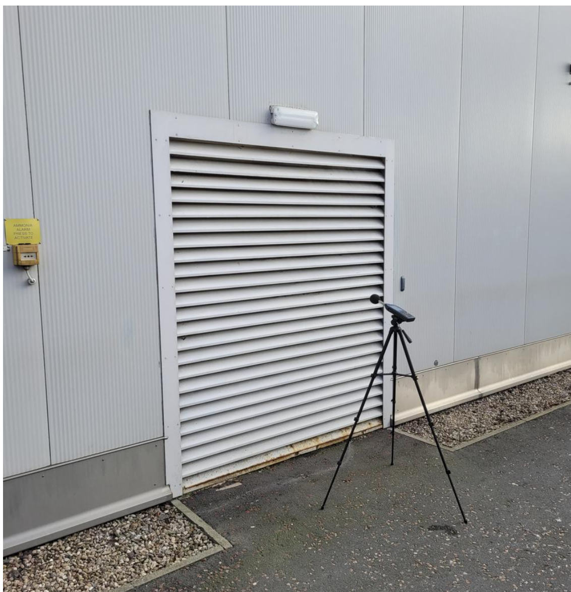
Figure D4: Ammonia Plant Room
