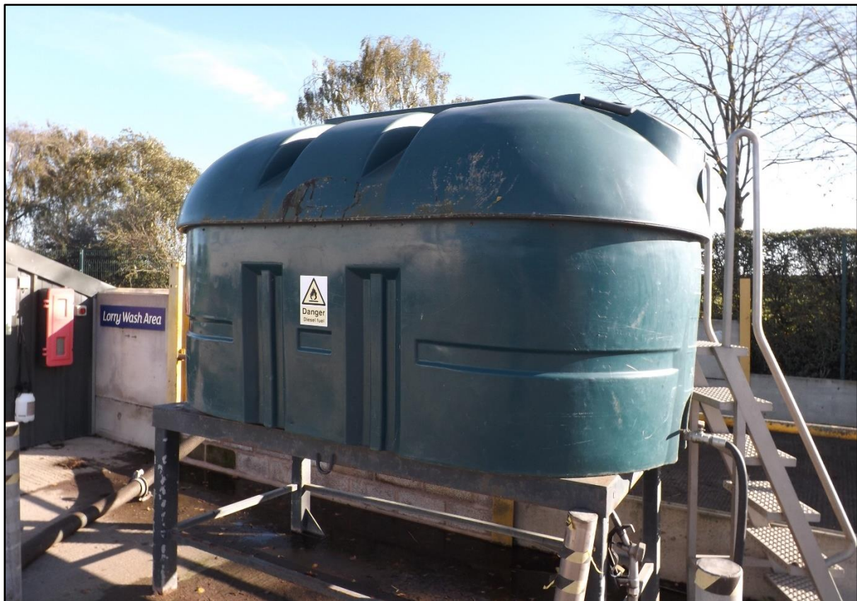
Figure 6.1: Double Skinned Tank
