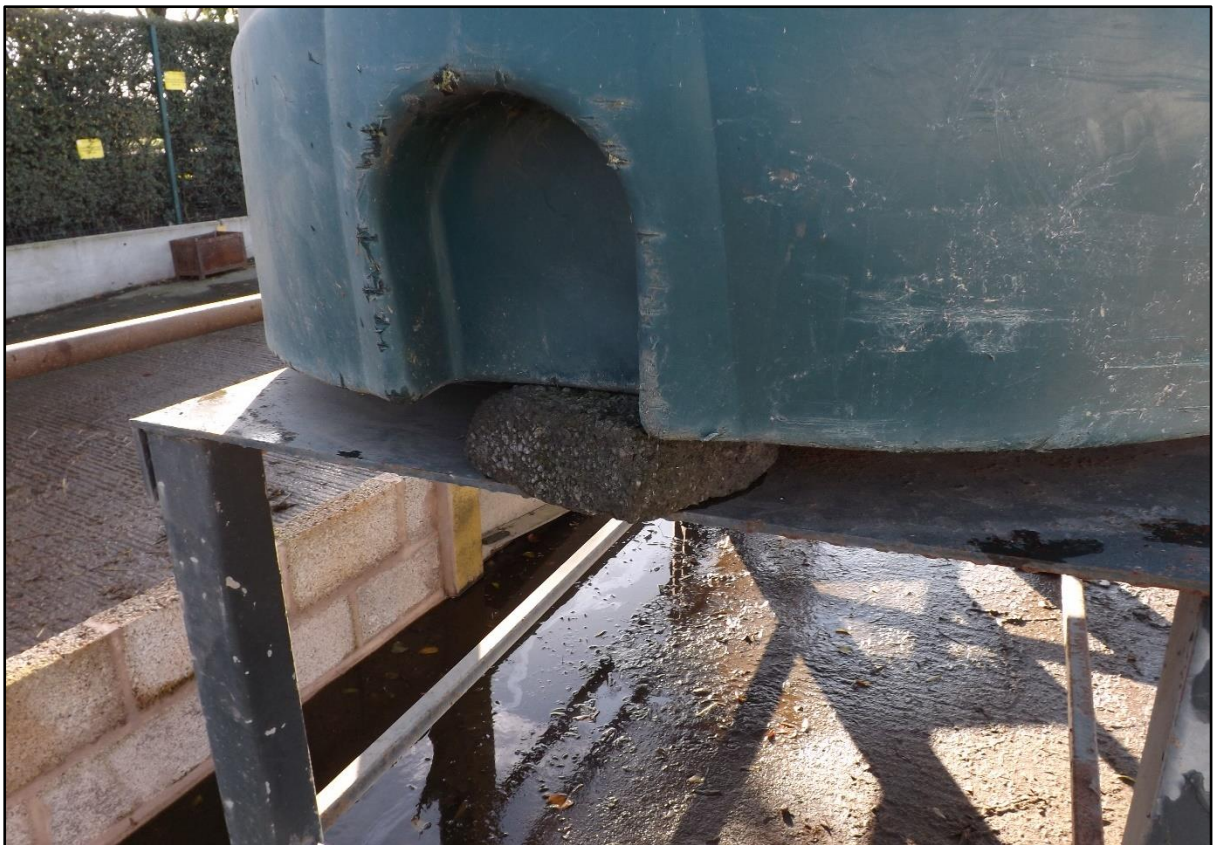
Figure 6.3: Concrete Block Beneath Eastern End of Structure
