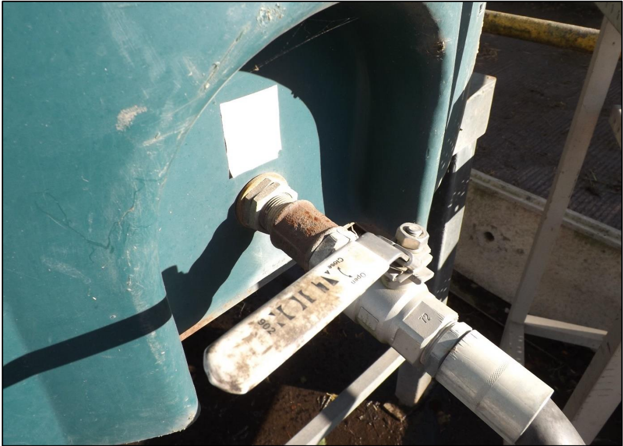
Figure 6.2: Tank Outlet Pipe and Valve
