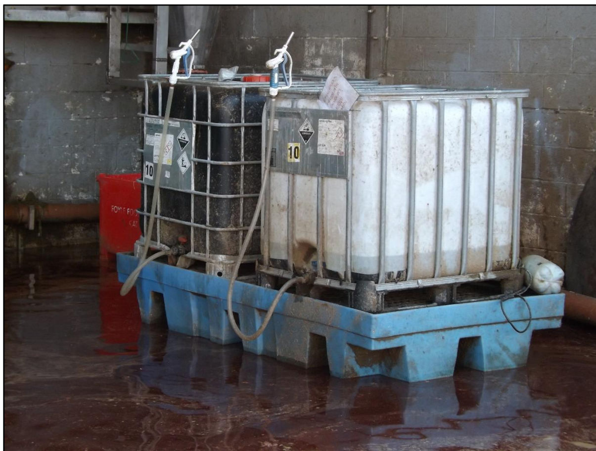
Figure 4: Double IBC Bund
