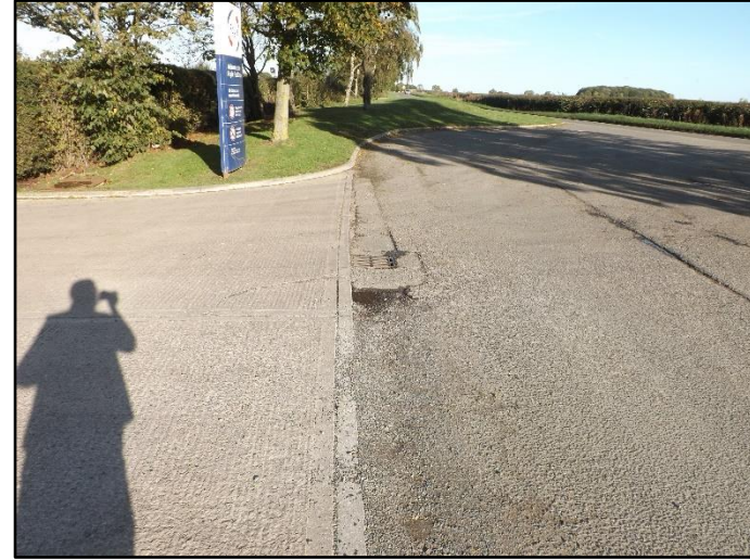
Figure D.2: Six Hills Ln Surface Drain
