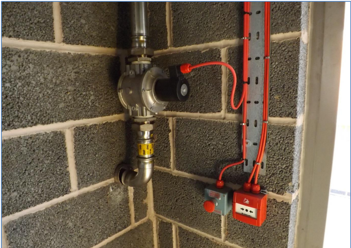
Figure 7.3: LPG Supply Pipe and Emergency Shut-off – Internal
