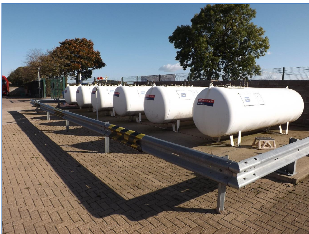
Figure 7.1: LPG Storage Tanks
