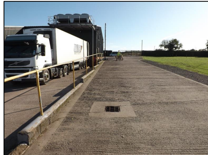
Figure 8: Clean Yard – Poured Concrete
