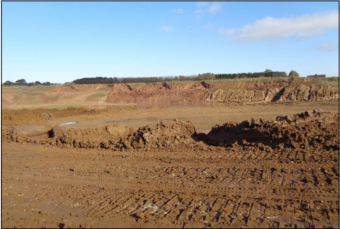
Photo 9. Surface erosion Phase 10 east slope.
