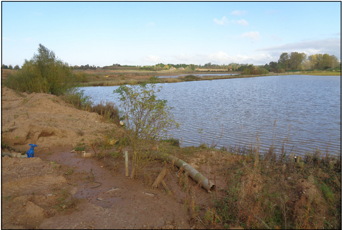
Photo 2. View of Silt Lagoon No.1, looking north.
