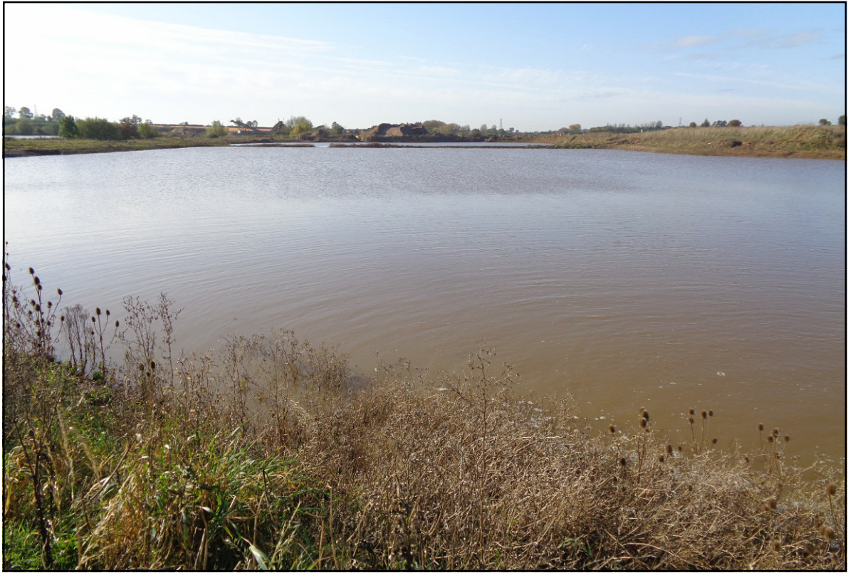
Photo 3. Recently constructed silt lagoons.
