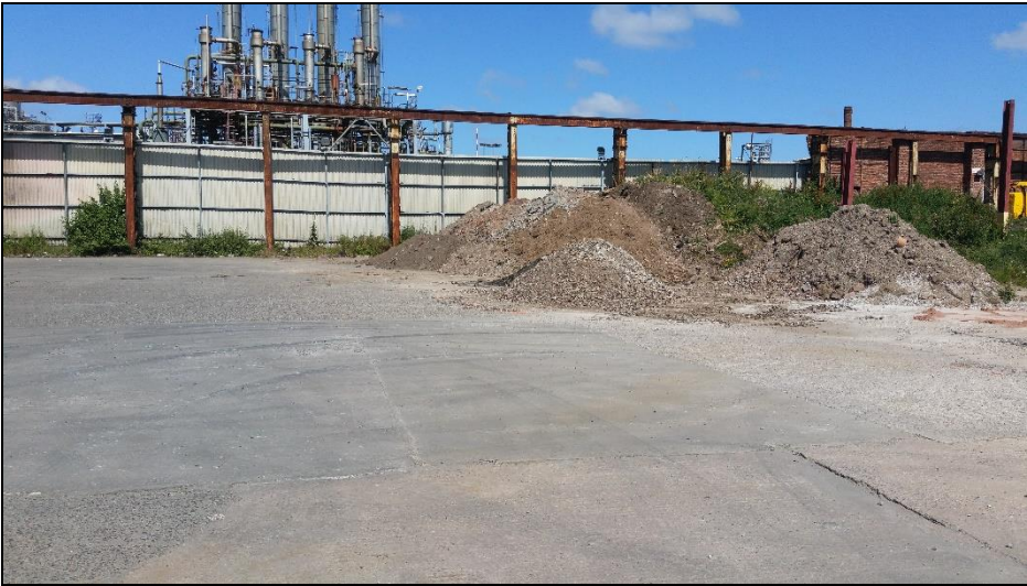
Photo 1. View from inside site looking West towards boundary with Veolia Solvent Plant beyond
