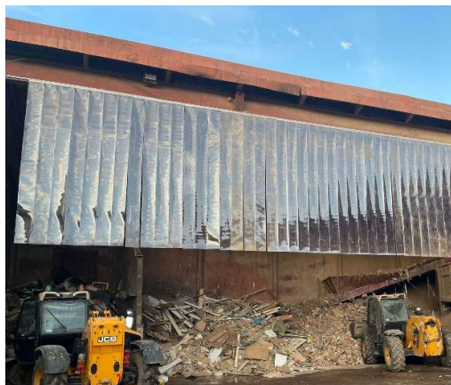
Figure 2 – View of existing building with Butcher Flaps
