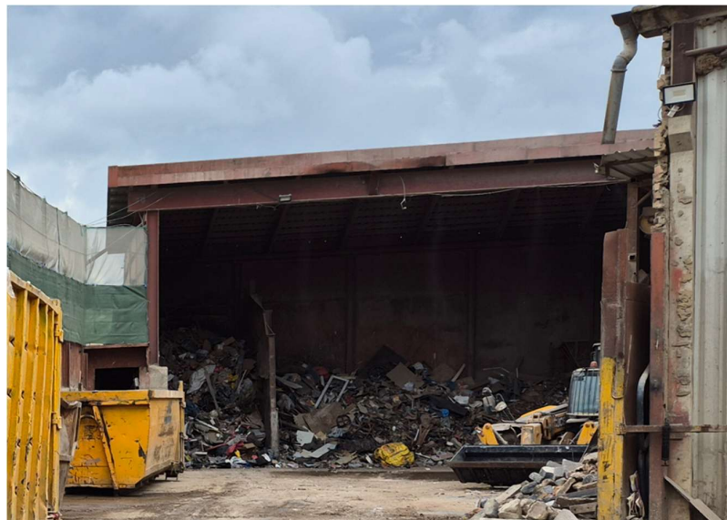
Figure 1 – View of existing building
