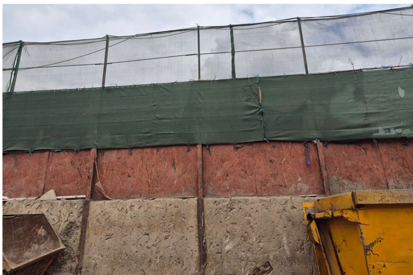
Figure 4 - Northern boundary – steel panels and litter netting
