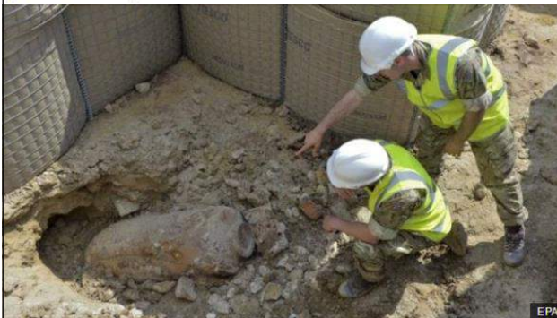
A 500lb World War Two bomb found on the site of a former school in Bath has been defused and made safe.
