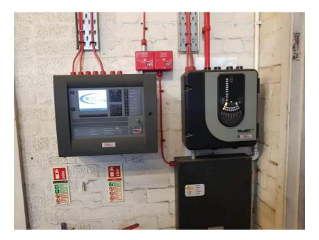
The battery treatment facility has a FAAST aspiration fire detection system installed, installed by Rosse Systems. Rosse Systems hold the following accreditations:
