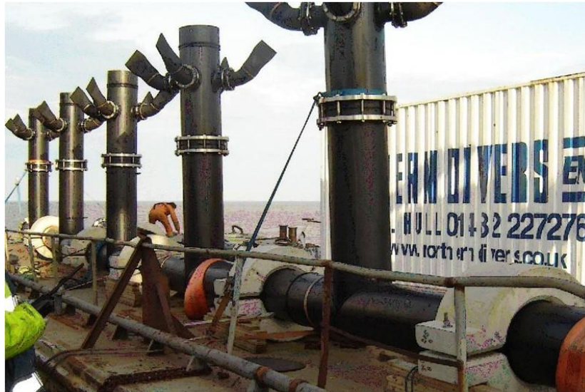
FIGURE 2-1: LINEAR DIFFUSER DESIGN, ONLY TWO RISERS OPERATIONAL (8 PORTS)
