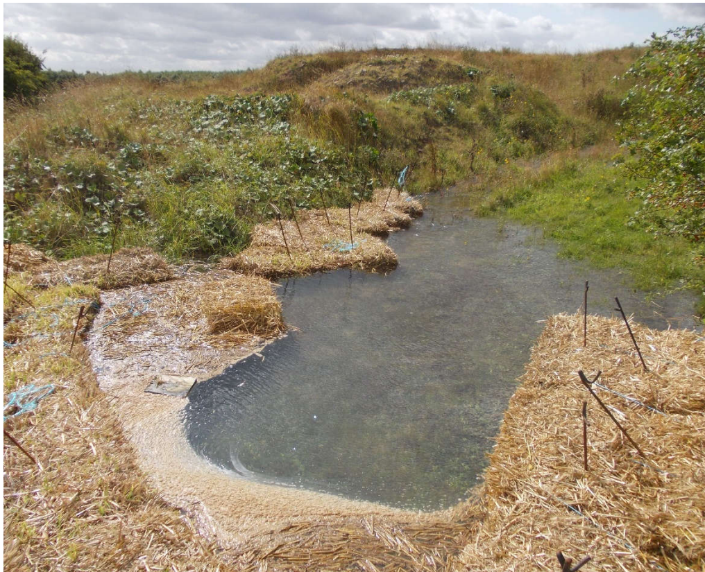
Photo 05: Straw bales dissipating water below discharge point
