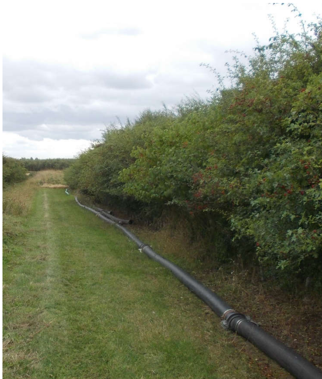
Photo 03: Discharge pipeline along compound boundary
