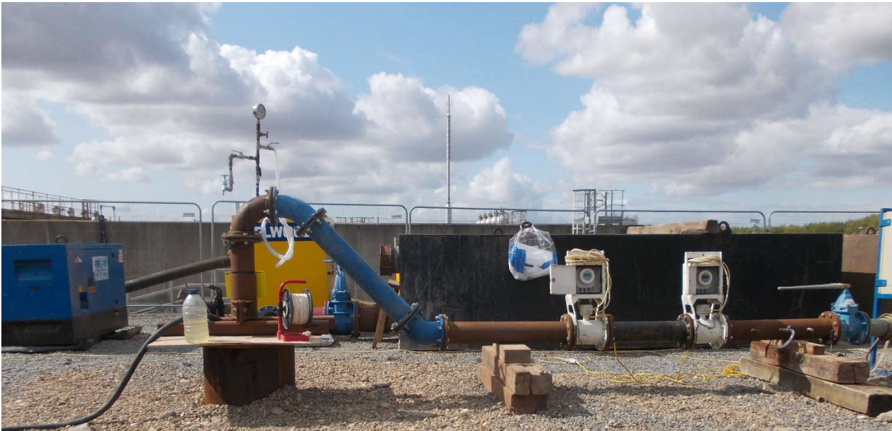
Photo 01: Abstraction borehole showing rising main and in-line flowmeters
