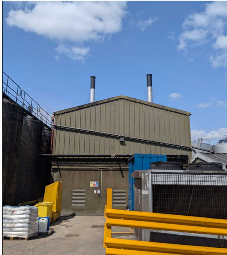
Figure 1: Emission Stacks from the boilers, in situ with neighbouring tanks.
