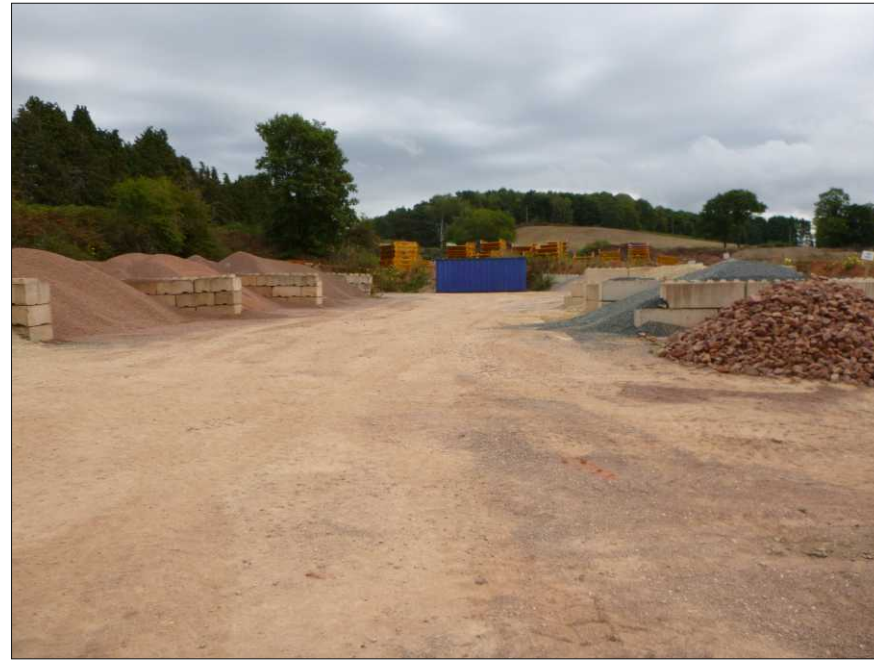
Photograph 2: Showing the bare ground of the worksite.
