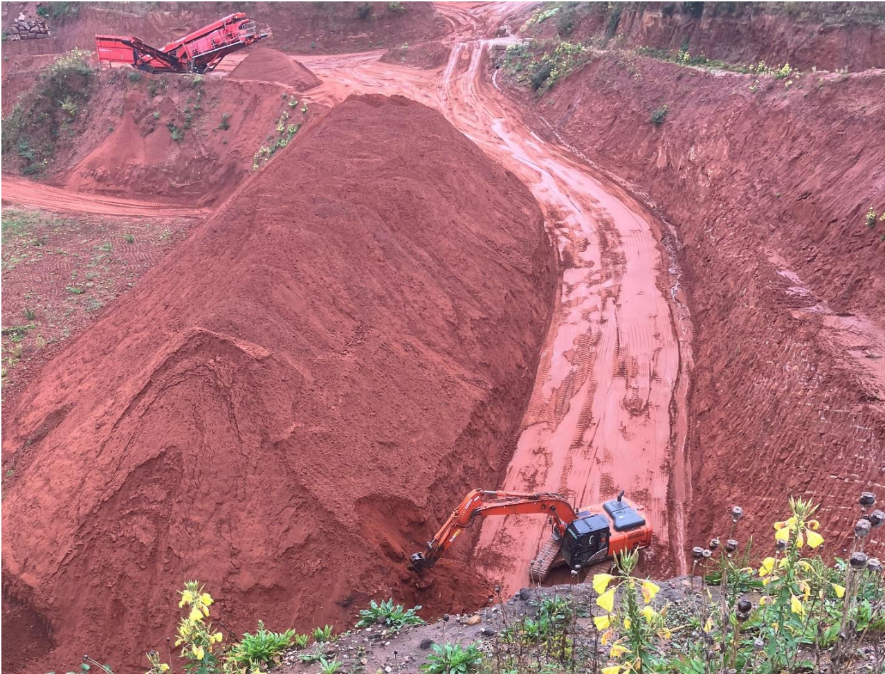
Figure 5.2 Surface Water Drainage (Ditch to Right of Road where Excavator Working)
