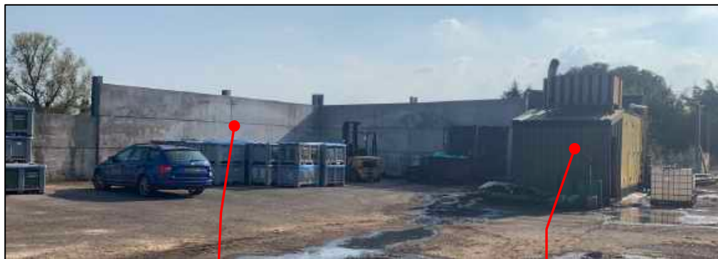
3.6m high concrete wall CHP unit/control room
