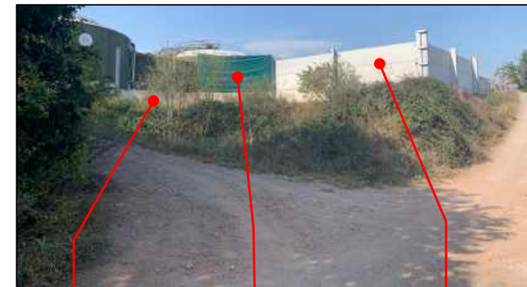
1 – 1.2m high concrete wall Lightweight screen with cooling fans/ CHP behind 3.6m high concrete wall
