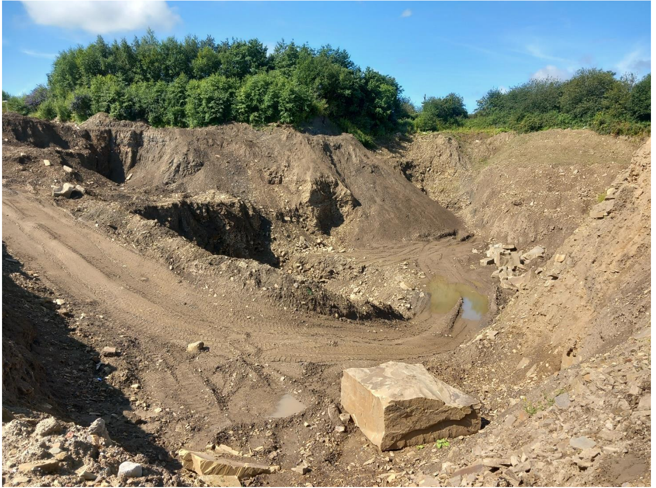
Photograph number 9 shows the small void recovery area to the west. The area is still being extracted but this is anticipated to cease before the deposit recovery permit is issued.
