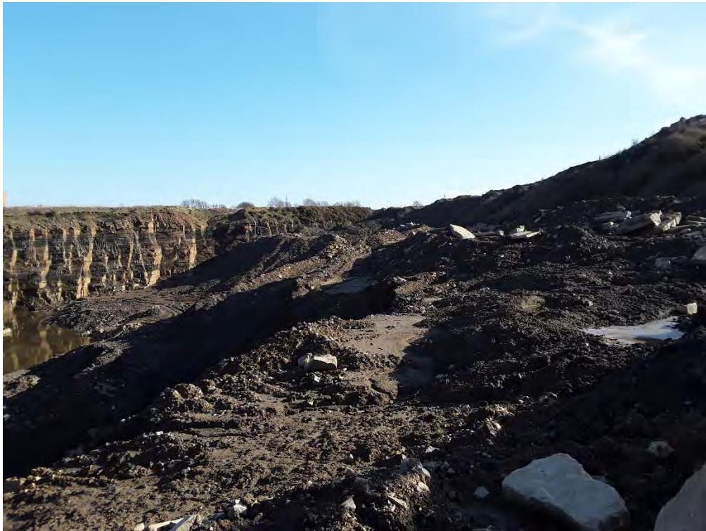
Photograph number 3 & 4 showing the quarry overburden and mining by-product stockpiles to be used as part of the fill operation as per the requirement of the planning consent
