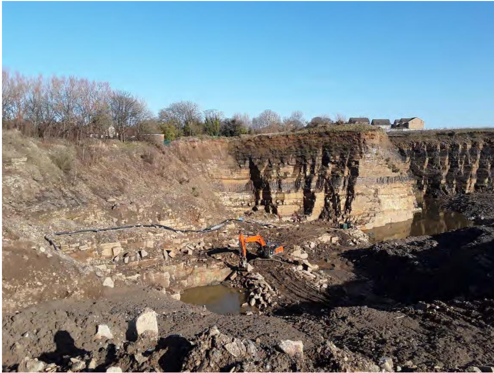
Photograph number 1 showing the northern face of the large void recovery area with sumps to collect surface water runoff for use on site.
