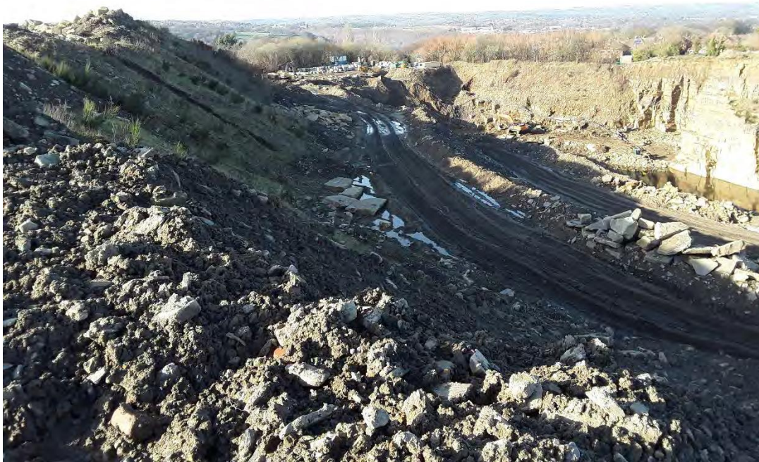
Photograph number 7 showing the berm bench placed in mudstone to support the minerals tip and access into the main void recovery area.
