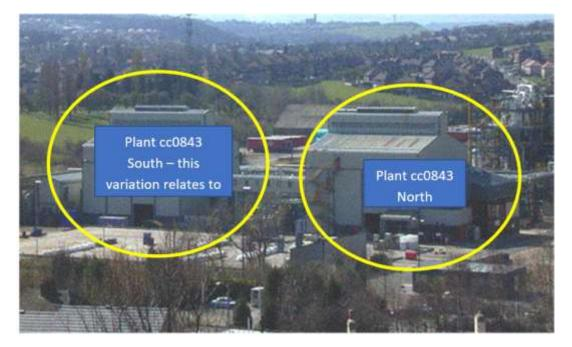
The proposed process in Plant cc0843 will be a manufacturing process to produce an insecticide active ingredient (AI), SYN547407. This AI is already made at another plant (cc0868) on site in smaller quantities and this change will allow the scale up of production of this AI by modifying an existing plant.
