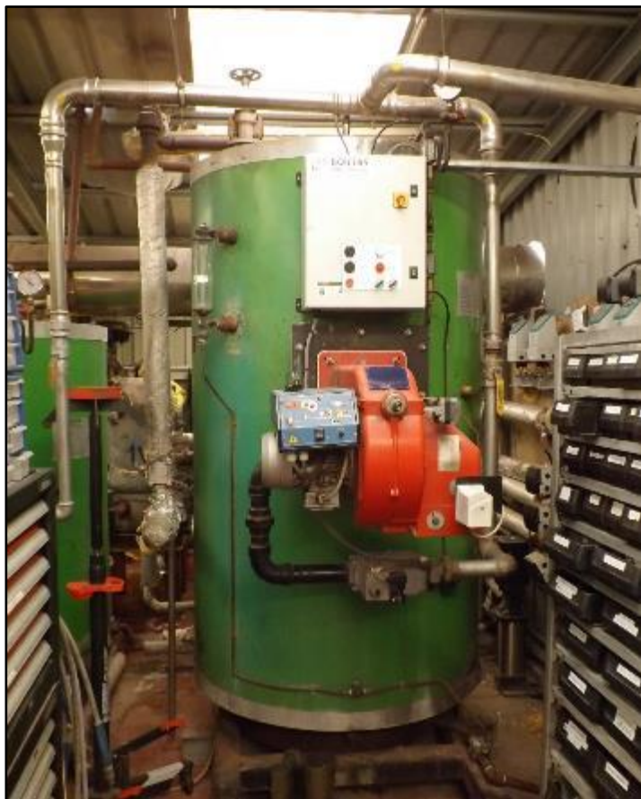
Figure 3.1: Steam Boiler Layout (B-1)
