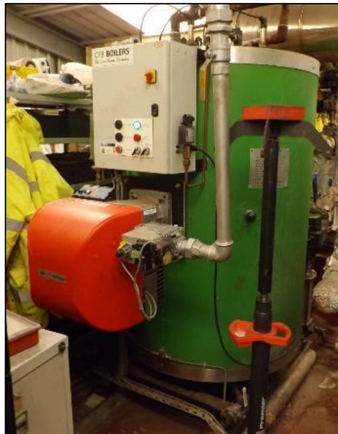
Figure 3.2: Steam Boiler Layout (B-2)
