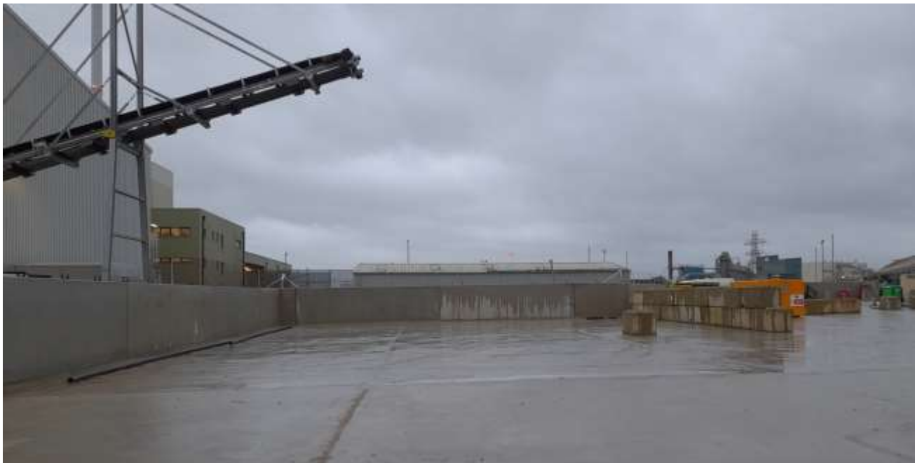
Figure 6. Plant Exit Conveyor
