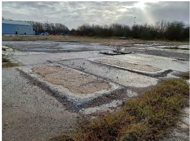
14.12.23 – Concrete pad near control room
