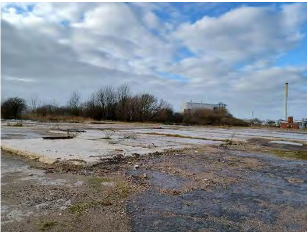
14.12.23 – Concrete pad for near autoclave area
