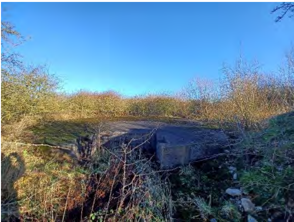
26.01.24 – View of circular concrete pad in west
