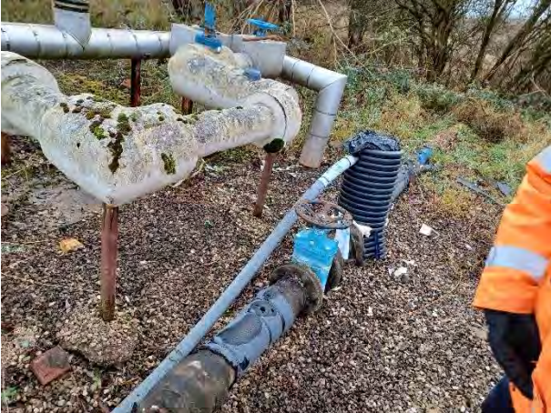
14.12.23 – Live water main off south boundary
