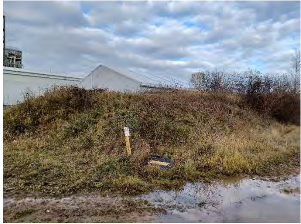
14.12.23 – Bunded material to prevent spillages from vinyl chloride tanks
