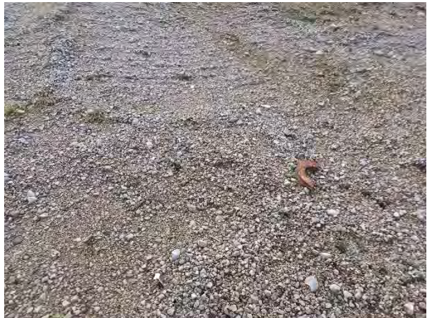
14.12.23 – Gravel site surface
