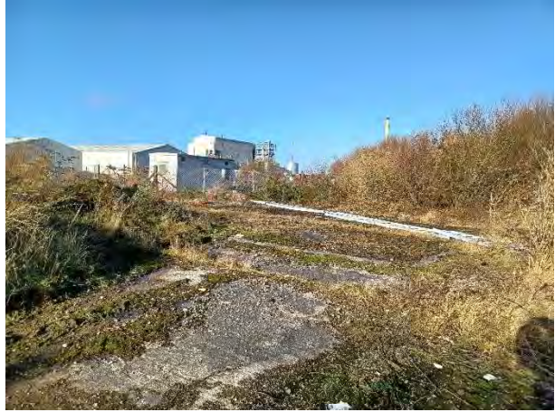
26.01.24 – Concrete pads in southeast
