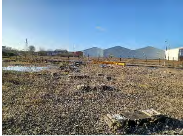
26.01.24 – View east across VCM off-loading area
