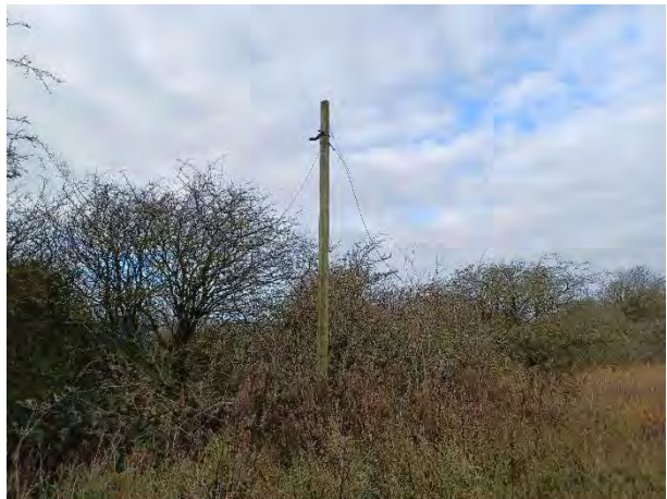
14.12.23 – Relict powerline pole located close to northern bank of Royles Brook.
