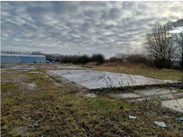
14.12.23 – Concrete pad in northwest of site
