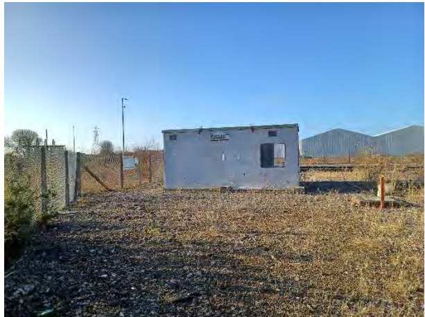
26.01.24 - VCM off-loading control room (east side)
