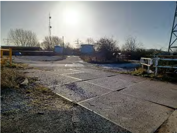
26.01.24 – Services access point in road
