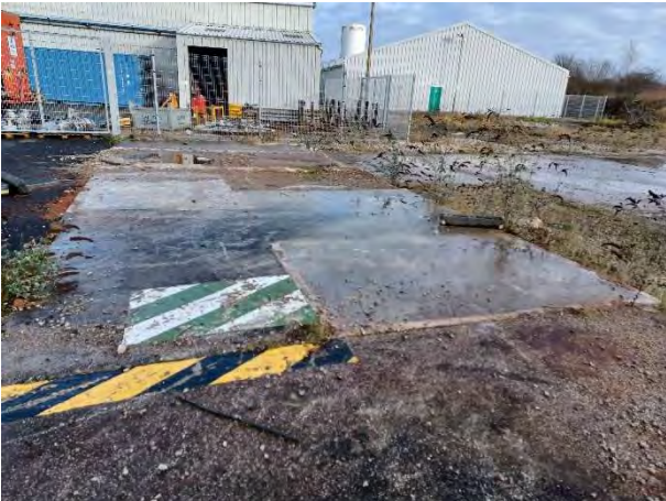
14.12.23 – Concrete pad for former cooling towers just off northwest boundary
