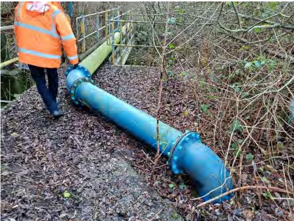
14.12.23 – Live water main crossing Royles Brook
