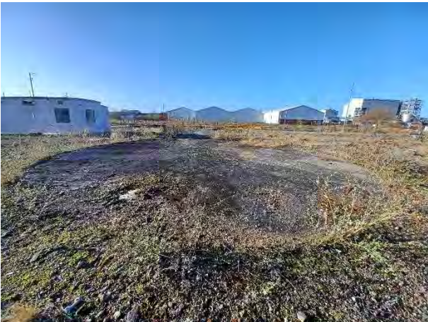
26.01.24 – Former VCM storage tank concrete pad
