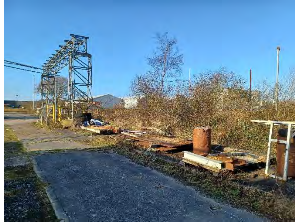
26.04.24 – View of southern boundary
