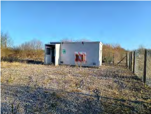
26.01.24 – VCM off-loading control room (west side)
