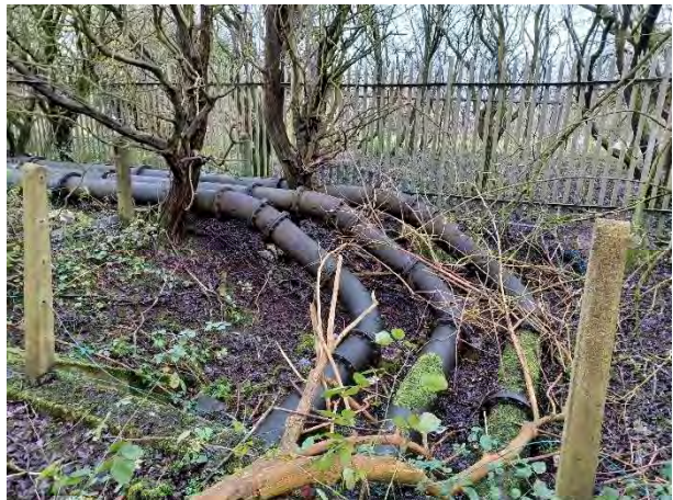
14.12.23 – Historical water / gas pipes
