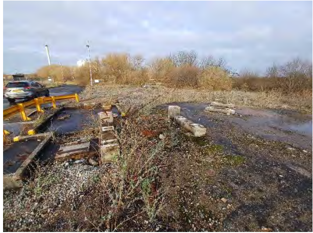
14.12.23 – Vinyl chloride drop off point (off-site)
