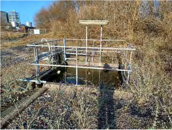
26.01.24 – Former spill drainage area (now used for surface water drainage)
