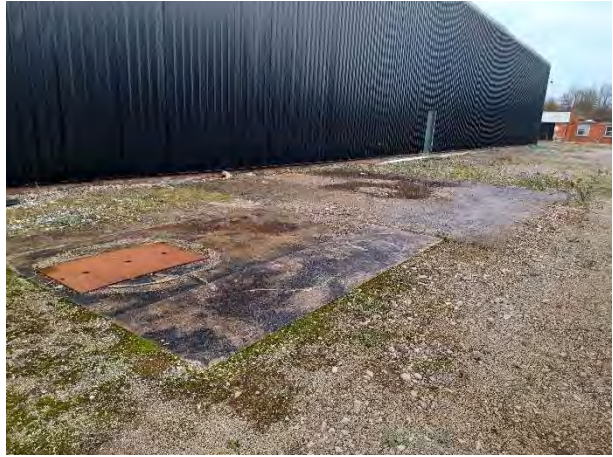
14.12.23 – Location of former chimney stack
