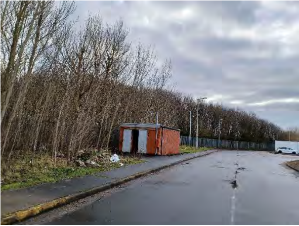
14.12.23 – Access road and off-site oil store
