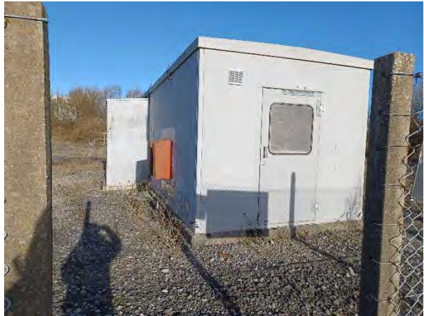
26.01.24 - VCM off-loading control room (south side)
