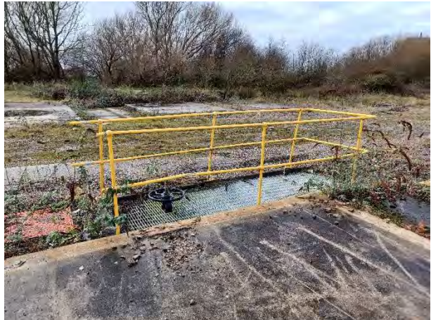
14.12.23 – Surface water drain access point near area of former mineralised water tanks
