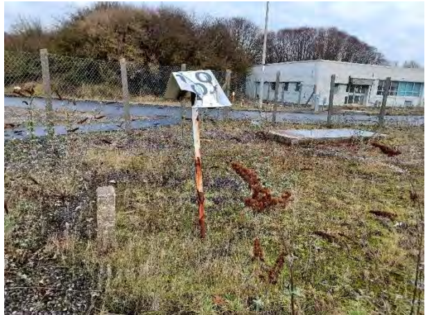
14.12.23 – Ethylbenzene pipeline marker post
