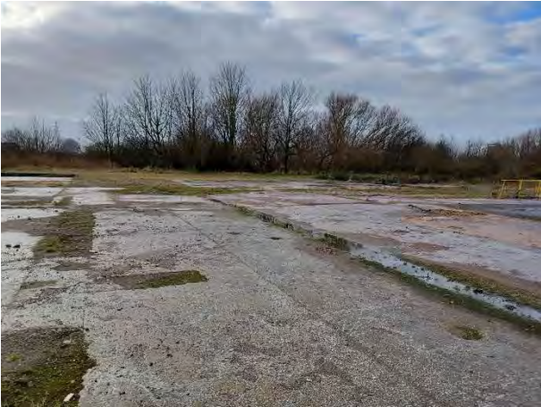
14.12.23 – View southwards across hardstanding in centre of site
