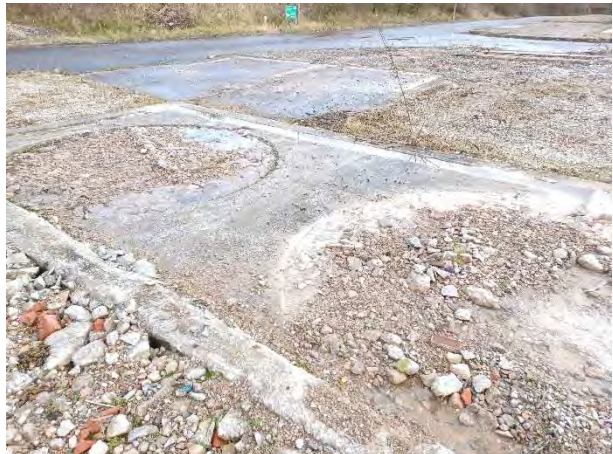
14.12.23 – Former location of effluent stirring tanks
