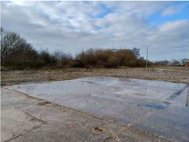
14.12.23 – Concrete pad near stripping column
