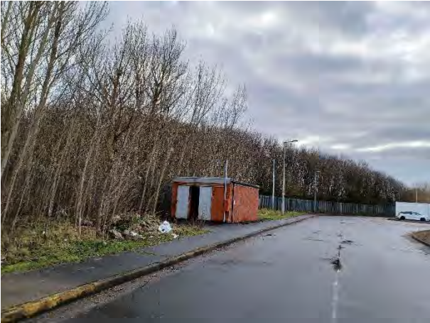
14.12.23 – Access road and off-site oil store
