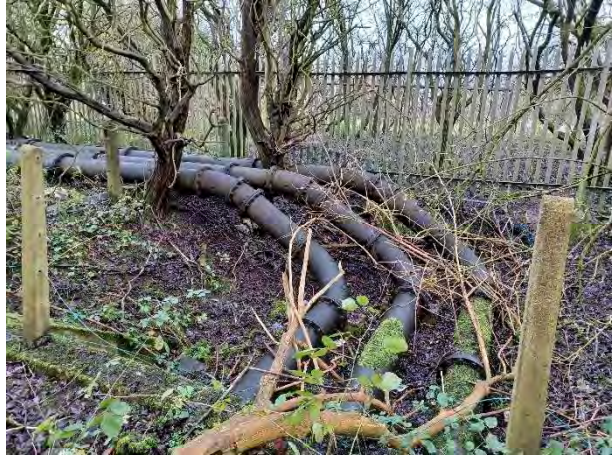
14.12.23 – Historical water / gas pipes
