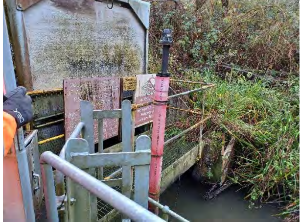
14.12.23 – Sluice gate on the southeast end of Royles Brook (off-site)
