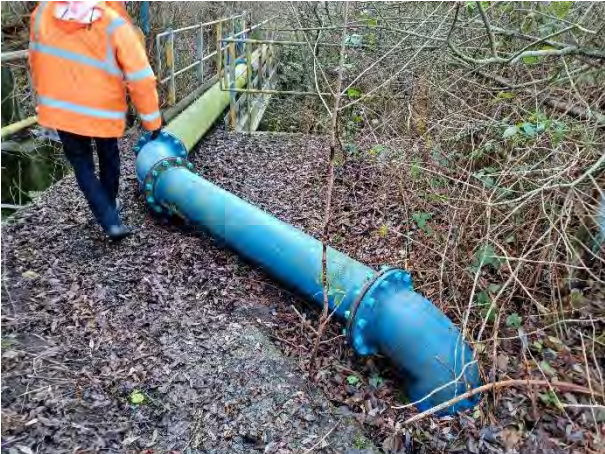
14.12.23 – Live water main crossing Royles Brook
