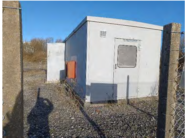
26.01.24 - VCM off-loading control room (south side)
