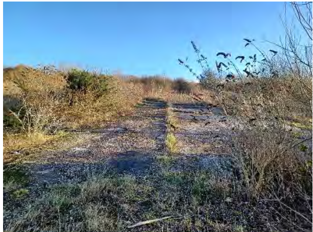
26.01.24 – Concrete pad in the south (unknown use)
