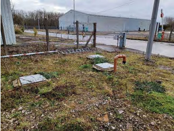
14.12.23 – Location of septic tank
