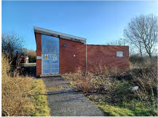
26.01.24 – West side of switch house to the south (off-site)
