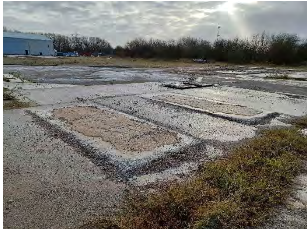
14.12.23 – Concrete pad near control room
