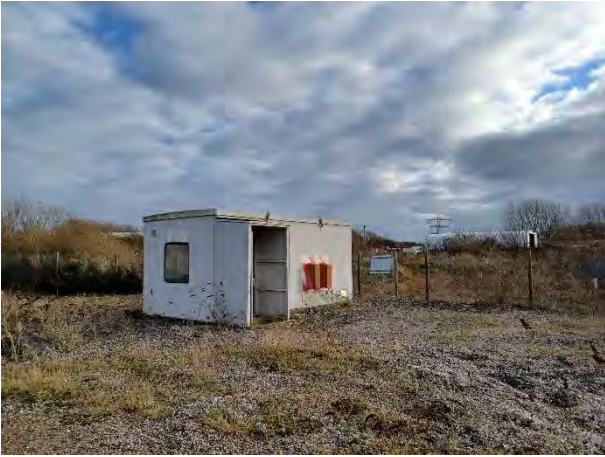
14.12.23 – Cabin at vinyl chloride drop off point
