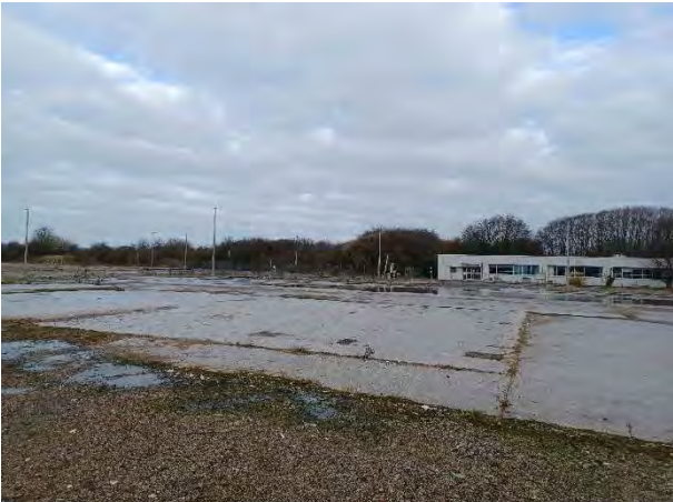
14.12.23 – Location of former control room
