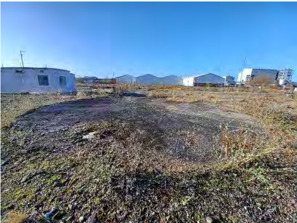
26.01.24 – Former VCM storage tank concrete pad
