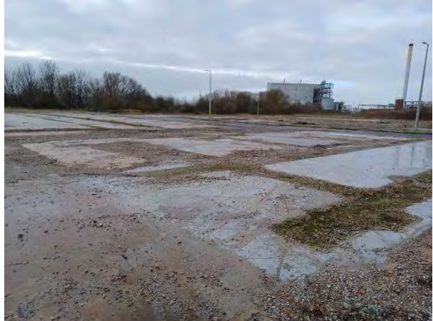
14.12.23 – Location of former latex tanks / autoclaves
