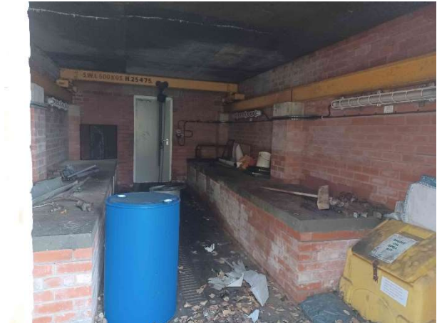
14.12.23 – Oil storage hut (off-site)
