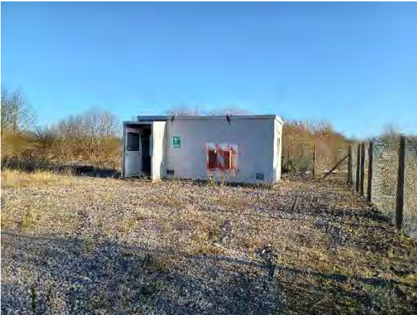
26.01.24 – VCM off-loading control room (west side)
