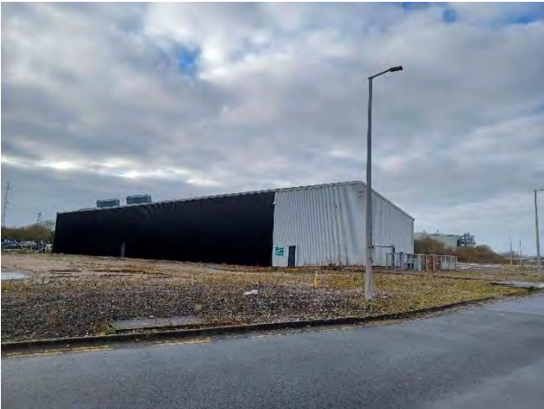
14.12.23 – View of existing business - Express Trade Frames (former boiler house)
