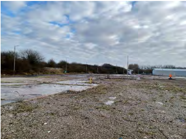
14.12.23 – View southeast from effluent treatment plant
