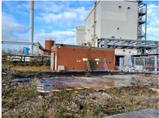
14.12.23 – 11kv switch house off northwest boundary
