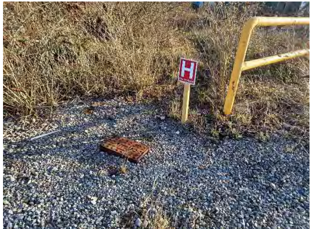
26.01.24 – Fire hydrant point connected to live water main
