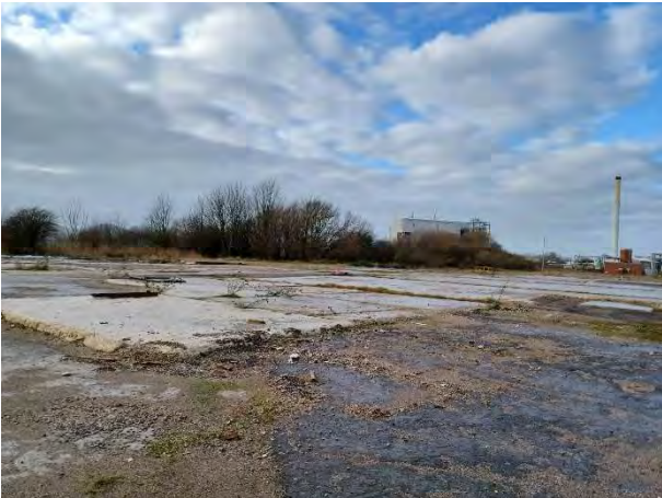
14.12.23 – Concrete pad for near autoclave area
