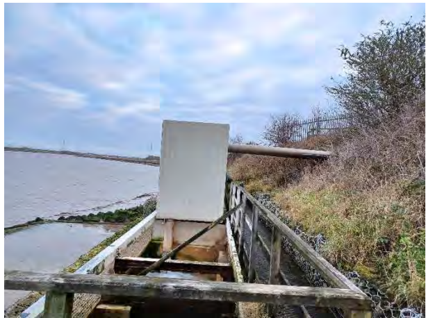
14.12.23 – Outfall drainage point (off-site)
