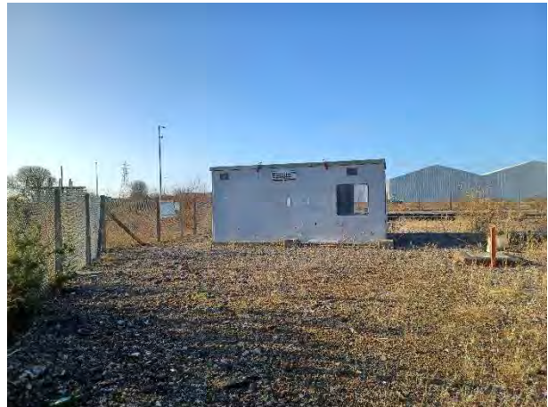
26.01.24 - VCM off-loading control room (east side)
