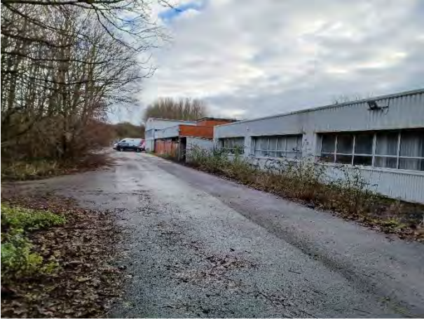
14.12.23 – Parking area/road to the rear of office building (off-Site)
