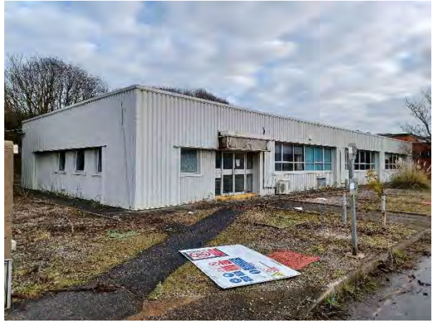
14.12.23 – Office building to remain
