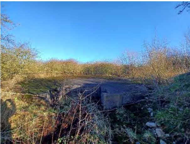
26.01.24 – View of circular concrete pad in west
