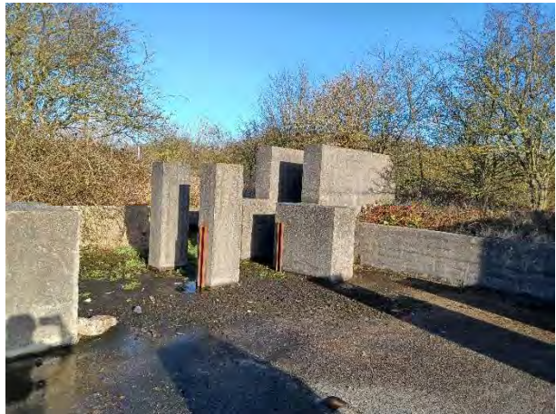
26.01.24 – View of unused foundation area on southern boundary
