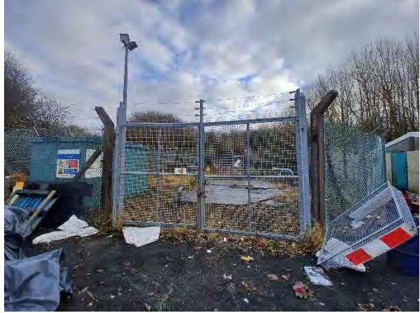
14.12.23 – Former high pressure gas main connection point (off-site)
