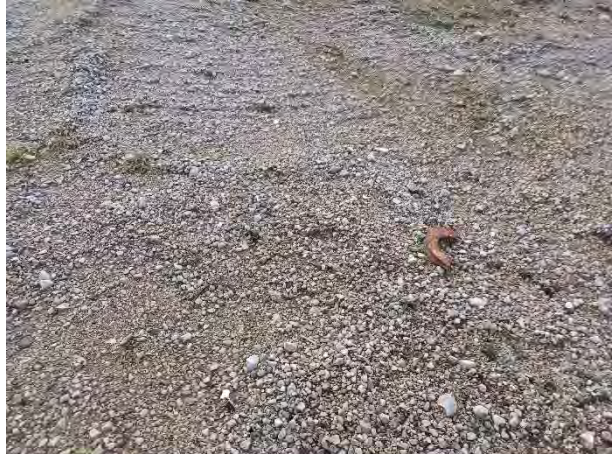
14.12.23 – Gravel site surface
