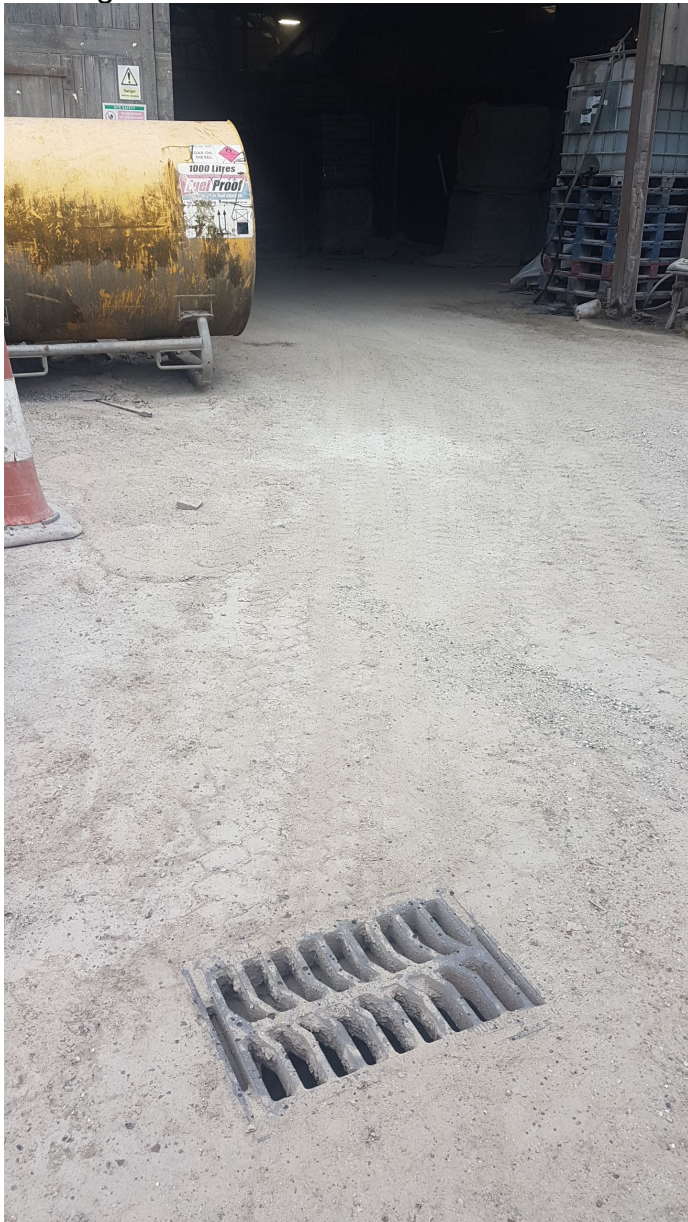
Photo 3: Surface water drain and concrete pad at entrance to main processing building
