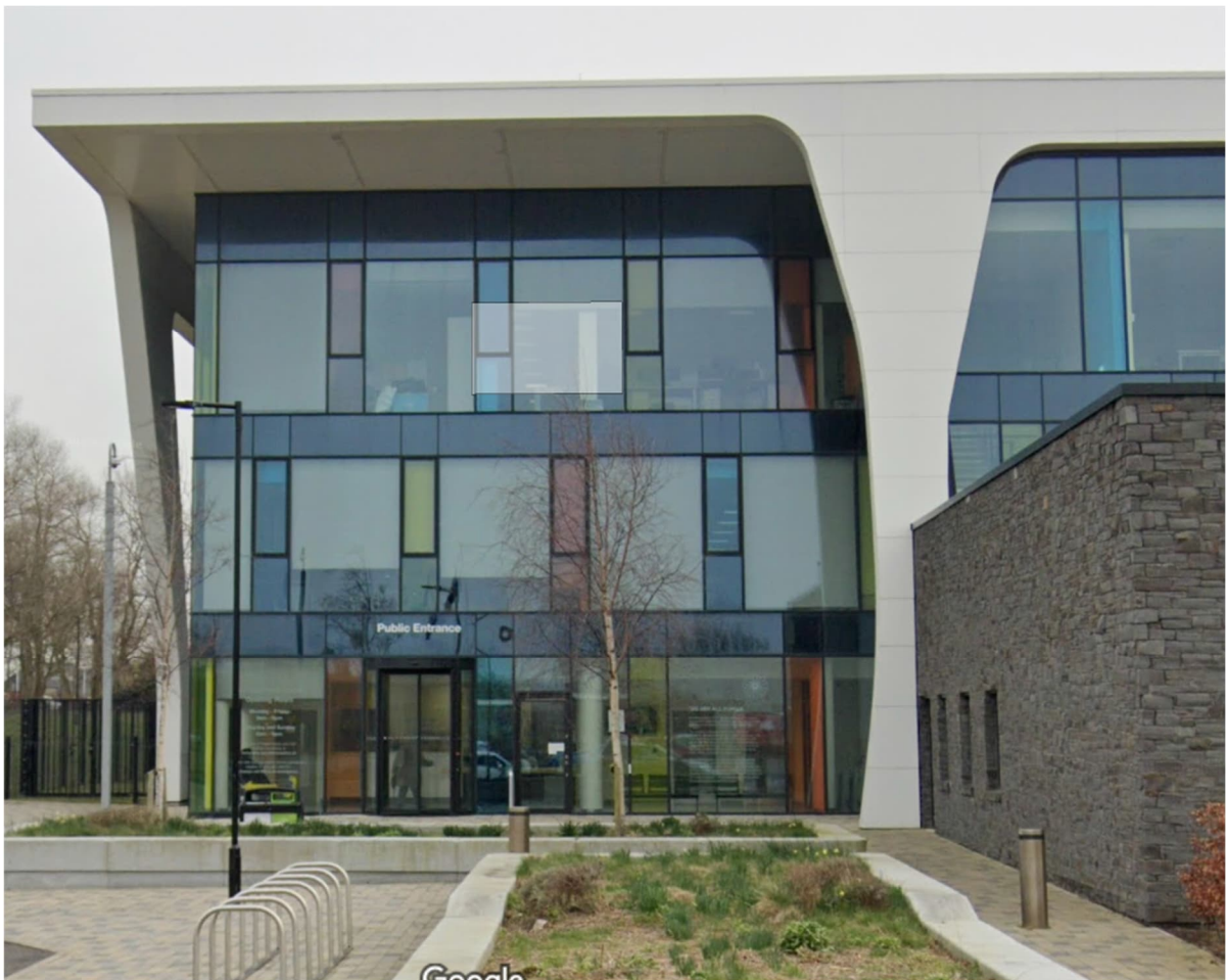
Figure 16 – Blackpool Police Headquarters building
