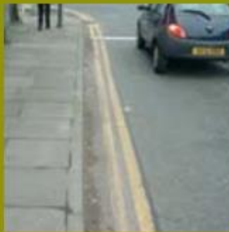
Grade C Widespread distribution of detritus with minor accumulations
