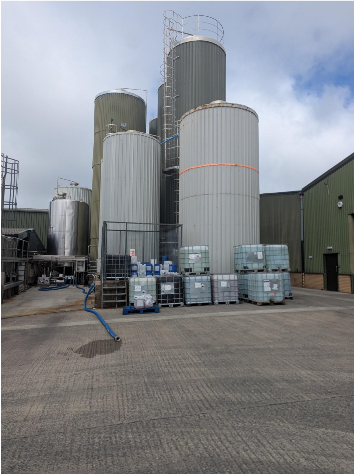
Photograph 4 – Silos and chemical storage on concrete surfacing
