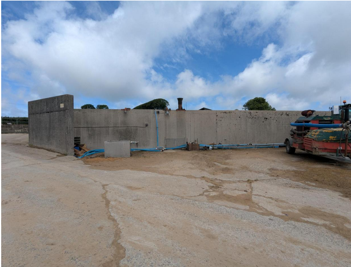
Photograph 15 – Concrete Dirty Water Tank (above ground) and adjacent yard
