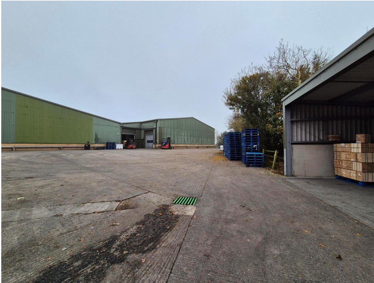
Photograph 8 – Site yard, looking to the north
