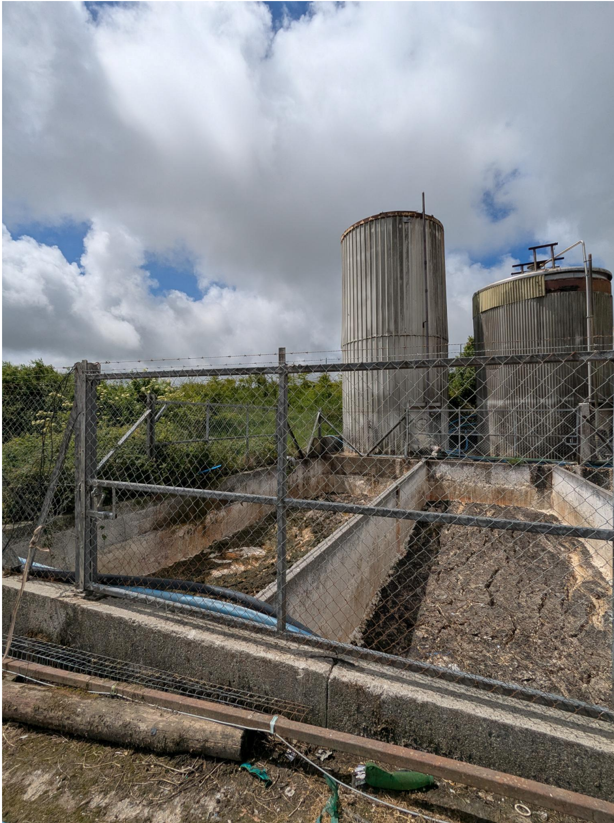
Photograph 14 –Concrete Dirty Water Tank (below ground) and Lactose Tanks
