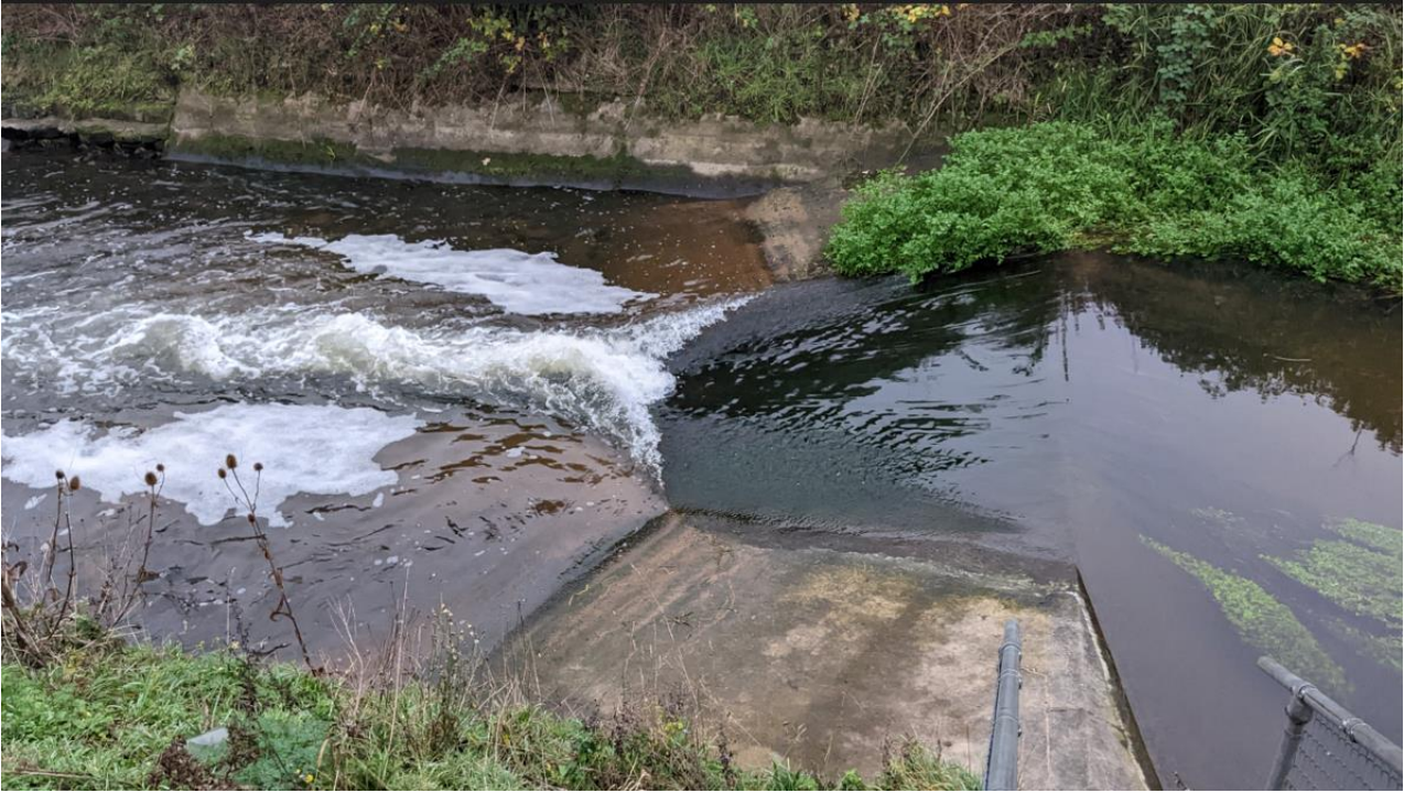
Figure 2-1: Weir, wingwalls and channel sides
