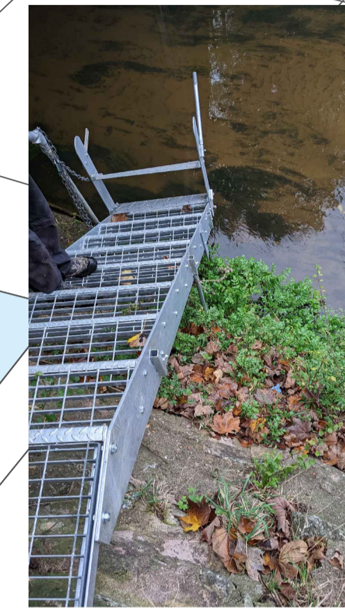
IMAGE 1 - STEPS IMMEDIATELY UPSTREAM OF BRIDGE (LEFT BANK)
