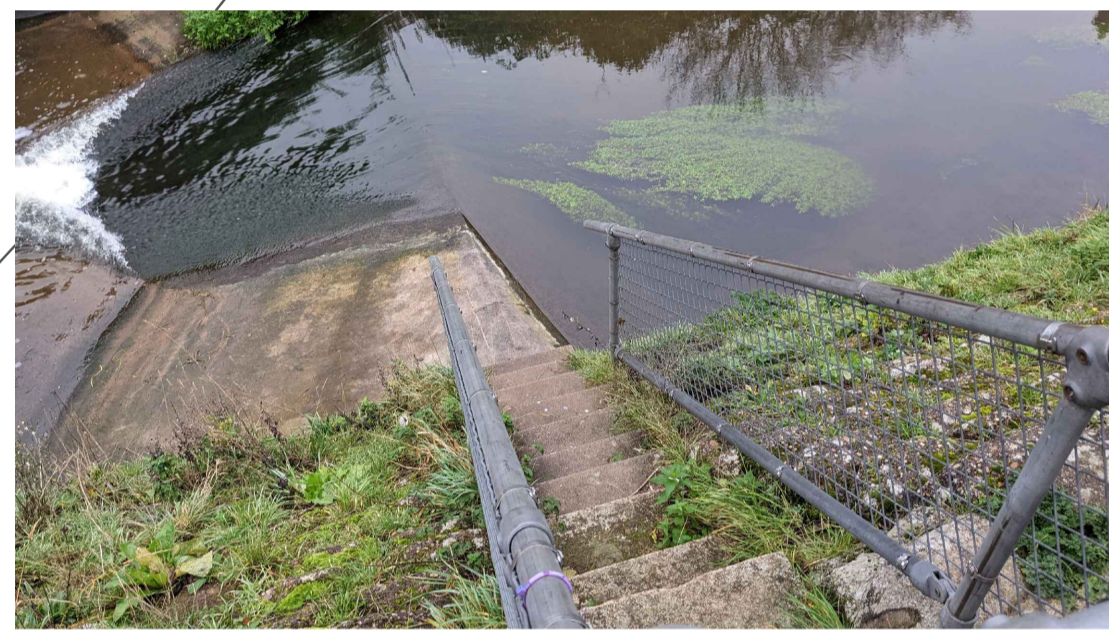
IMAGE 2 - STEPS AT WEIR
