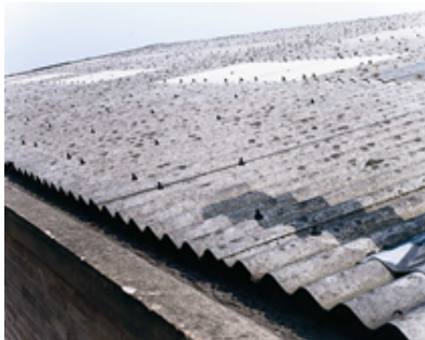
Asbestos Containing Roof
