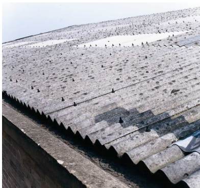
Asbestos Containing Roof
