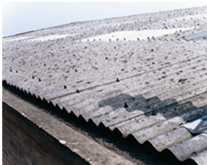
Asbestos Containing Roof
