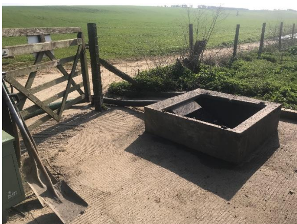
Plate 3. Concrete surround and impermeable pavement.
