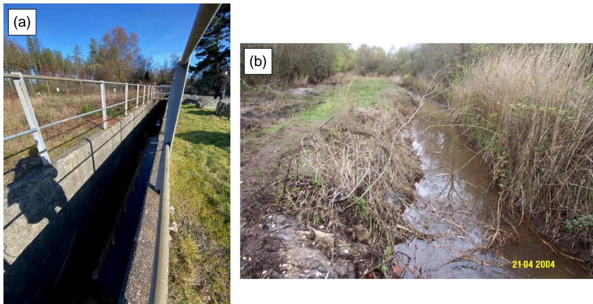
Figure 3.9: (a) Flume 1 (February 2024), which carries surface and ground water from the drainage network to a 1.2 m wide pipe under the railway line and into the Frome Ditch [36, Fig.1-4]. (b) The Frome Ditch in 2004, which carries water from Flume 1 and the culvert beneath the railway line to the River Frome (from the NRS IMAGES database).
