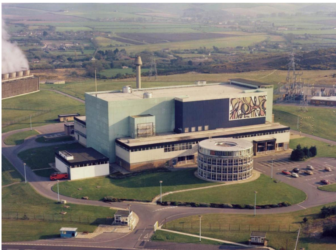
Figure 2.1: The SGHWR building (D60), cooling towers and electricity sub-station during its operational period.
