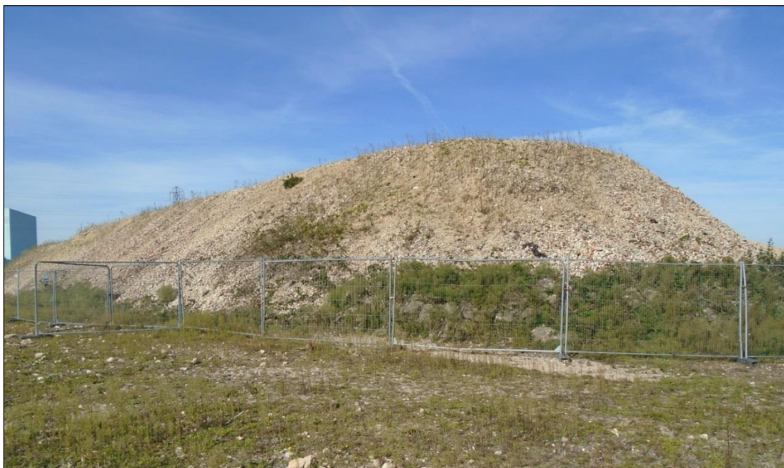
Figure 2.31: Main Rubble Stockpile (Stockpile 1) [99].
