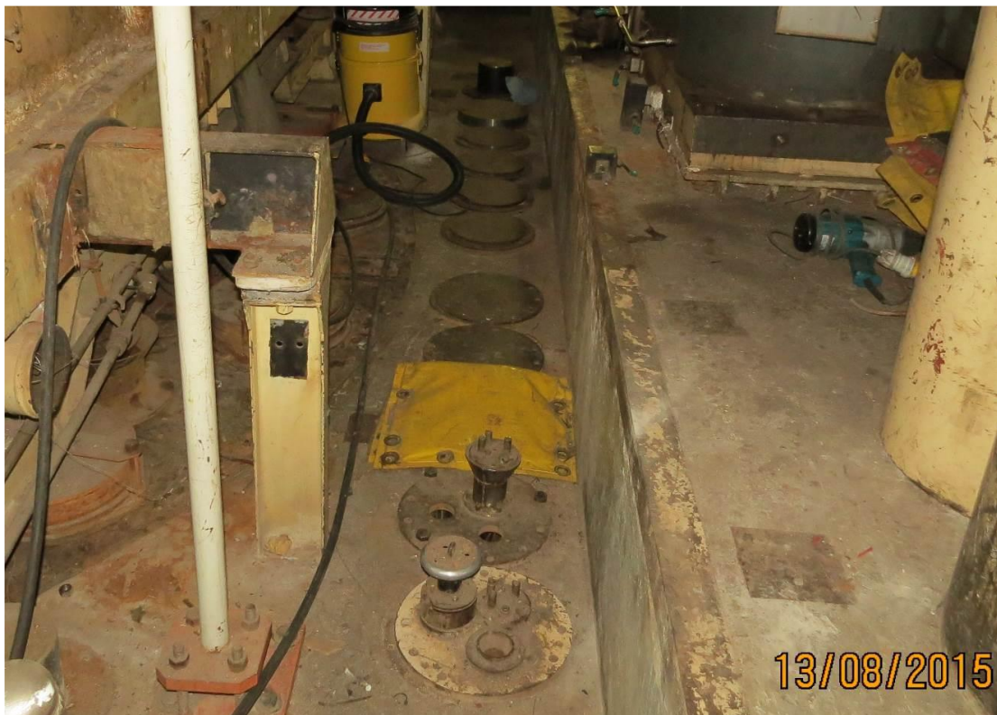
Figure 2.14: Image of the tops of the mortuary tubes taken in August 2015. Image looks north (closest visible mortuary tube is Z1); the top of the reactor is on the left. Mortuary tube Z3 is covered by a yellow square lead-filled blanket whose purpose is to shield the current contents; this will be removed as part of decommissioning [52].
