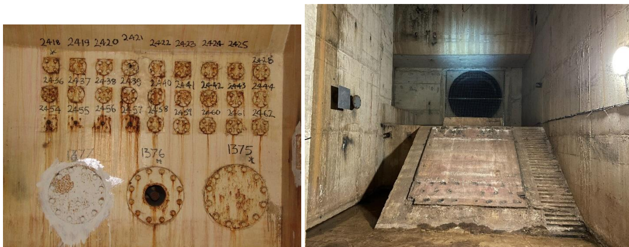
Figure 5.3: Examples of penetrations in the SGHWR below-ground structures, ranging from relatively small pipe openings (left) to large emergency cooling water mains (right).
