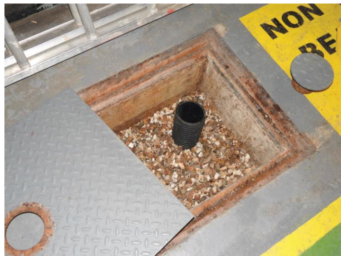
Figure A10: Typical manhole hatch above cofferdams. To be sealed as part of End State configuration.
