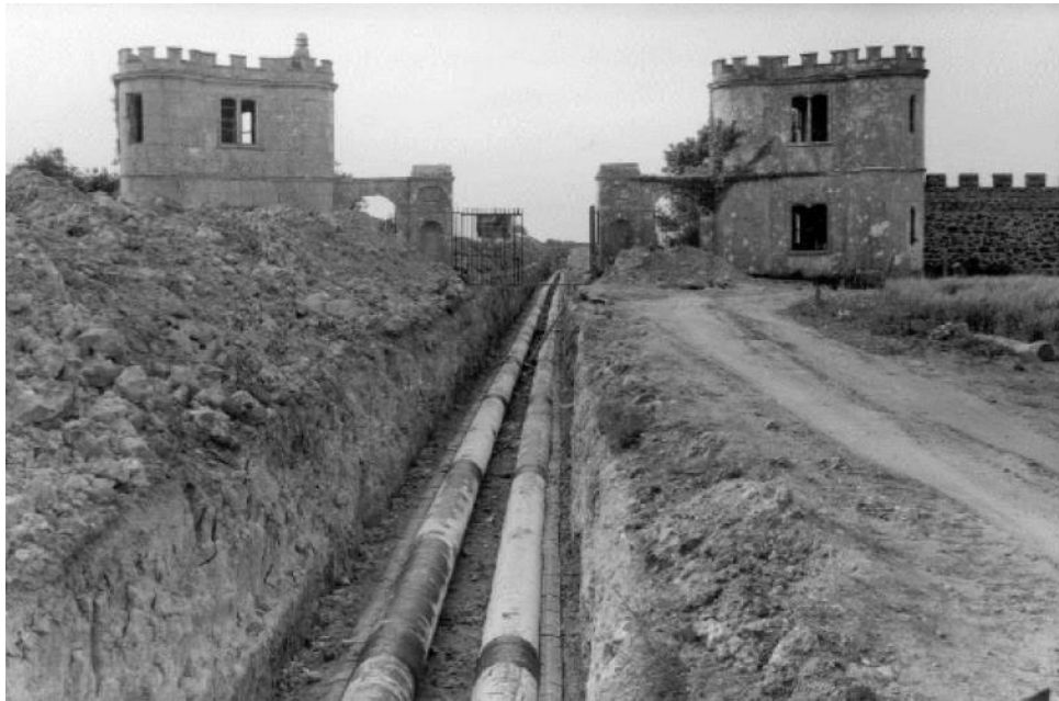
Figure 2.6: Image showing the construction of the Sea Discharge Pipeline and its route through the gates of Lulworth Castle [50, Fig.2.2].
