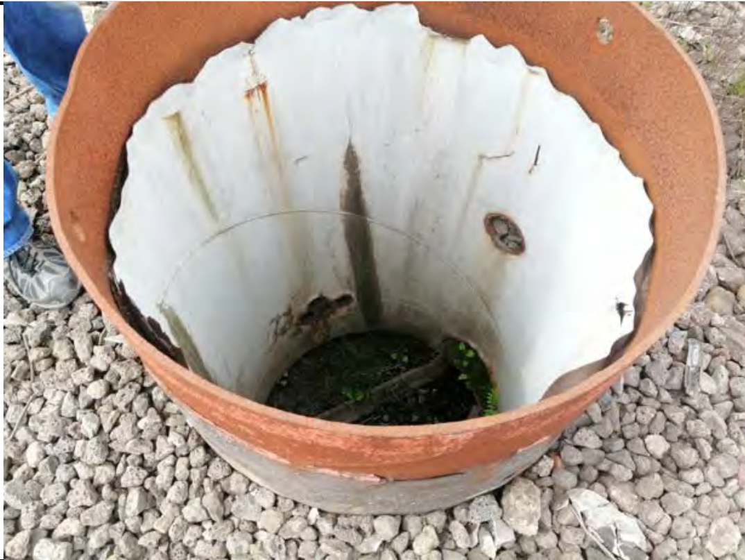
On site drain (1)
