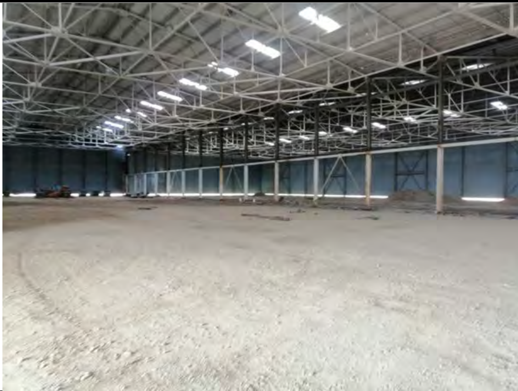
Inside the warehouse (Western area)
