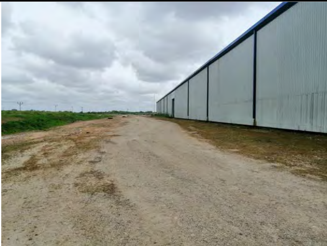
View from northwestern corner (Facing East)
