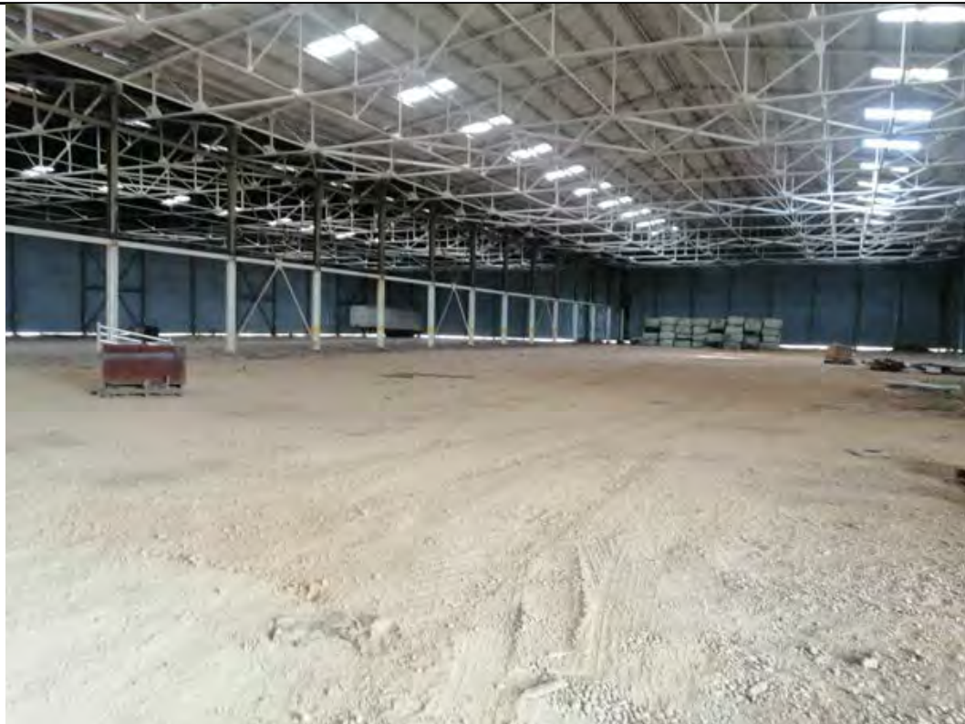
Inside the warehouse (Eastern area)
