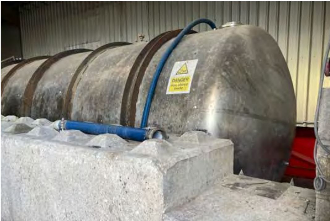
Photo 3: Lead sludge tank. This will not be used in the future process as battery breaking will become automated
