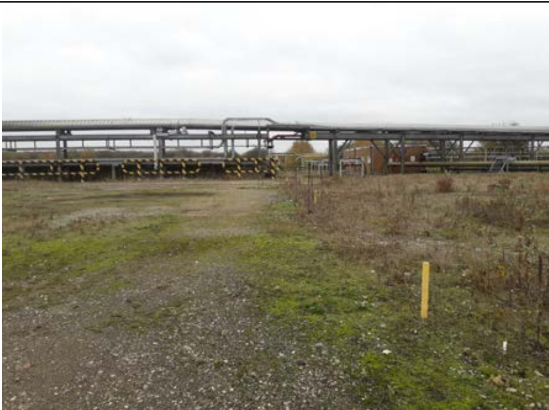
The southeast border of the site (Facing northeast)
