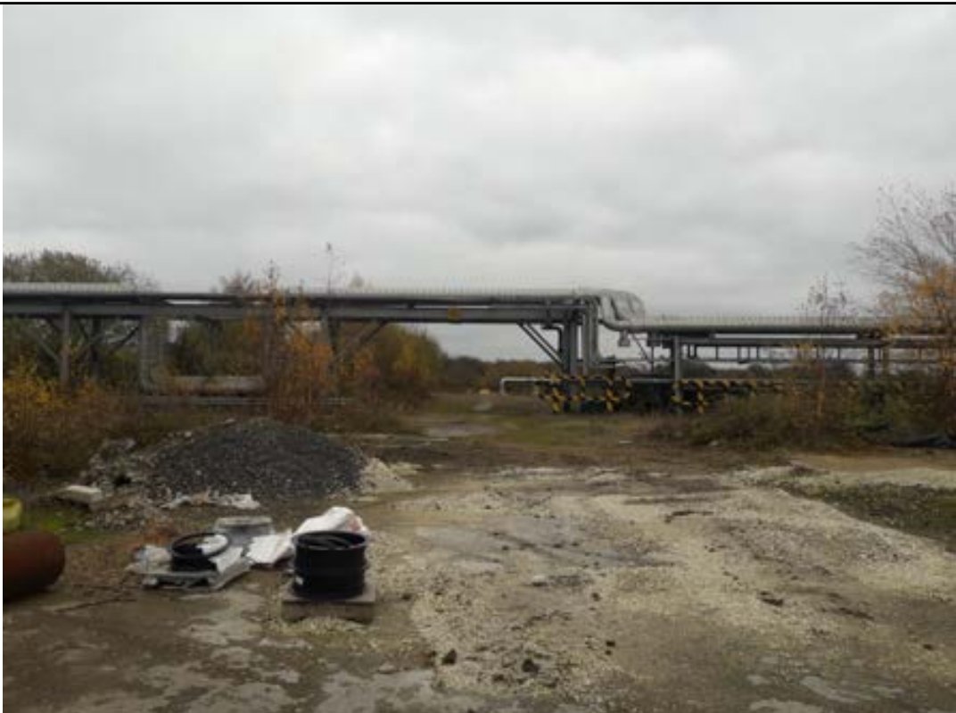
Facing northeast from the sites southwest
