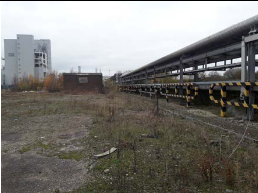
The east border of the site (Facing northwest)
