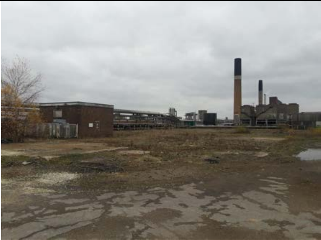
Facing east from the sites southwest
