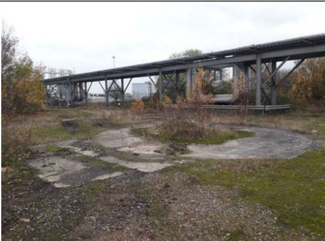
One of the tank bases
