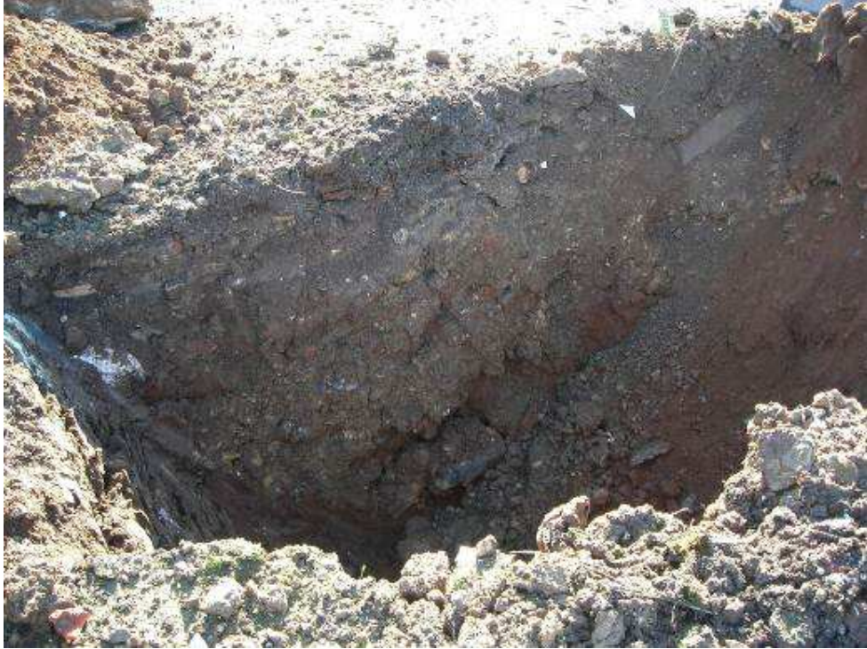
Detail of Trial Pit 3
