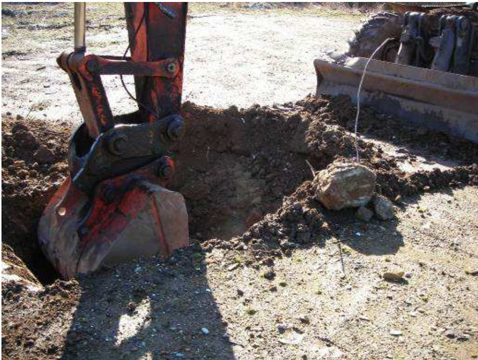
Detail of Trial Pit 4
