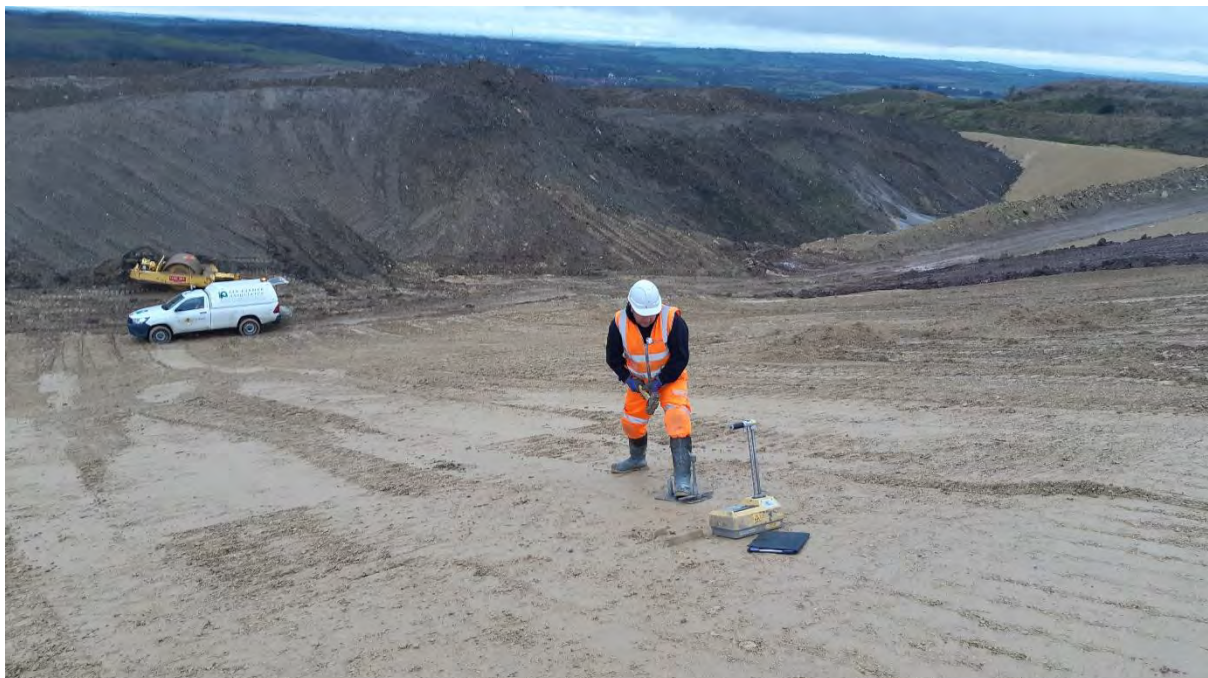
Nuclear Density Testing on north batter slope
