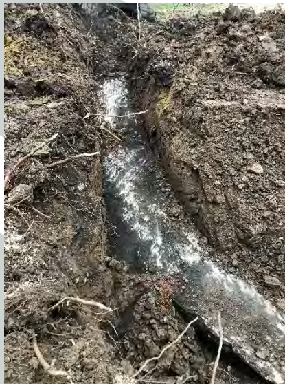
Photo No. 4 - 433550-003 Eastern Edge of Concrete
