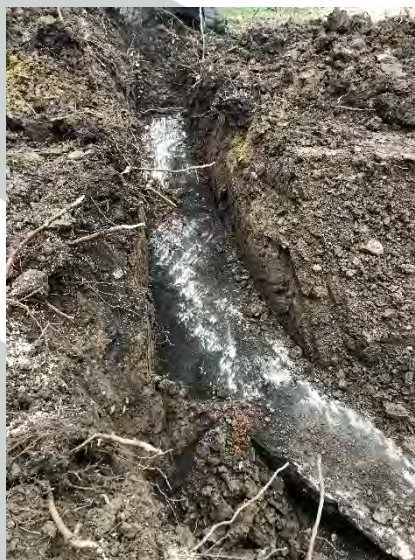
Photo No. 4 - 433550-003 Eastern Edge of Concrete
