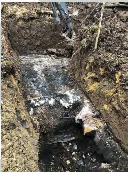
Photo No. 3 - 433550-003 Southern Edge of Concrete
