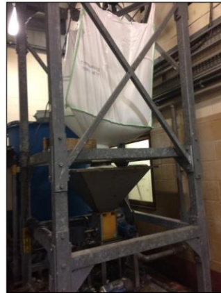
Figure 2: Polyelectrolyte hopper.
