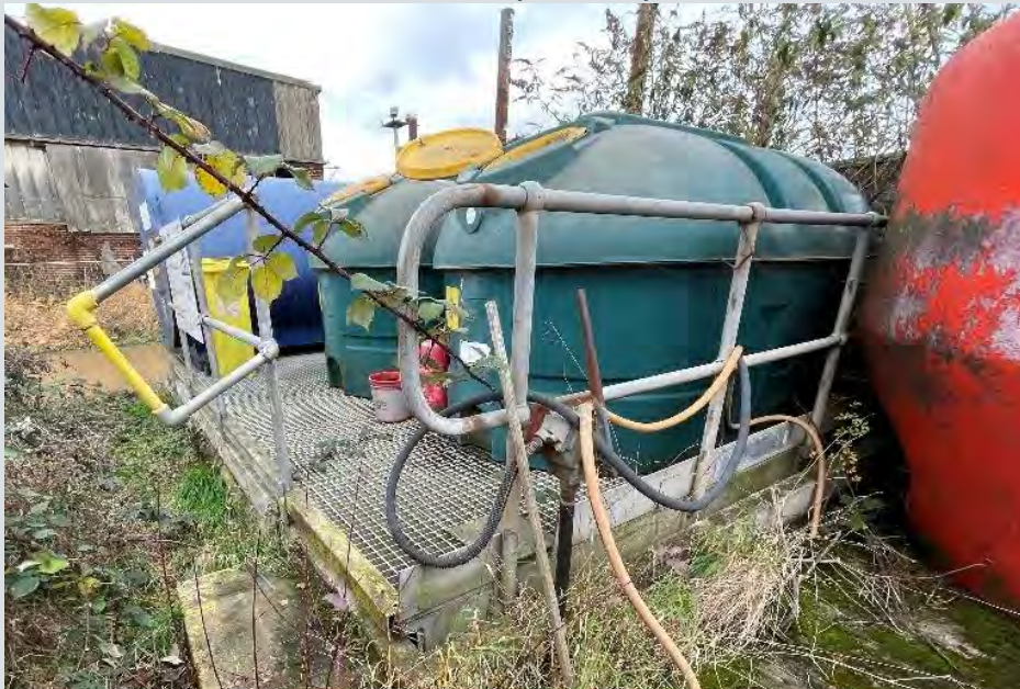
Plate 2.2 Above Ground Waste Oil Tanks (Source S2)
