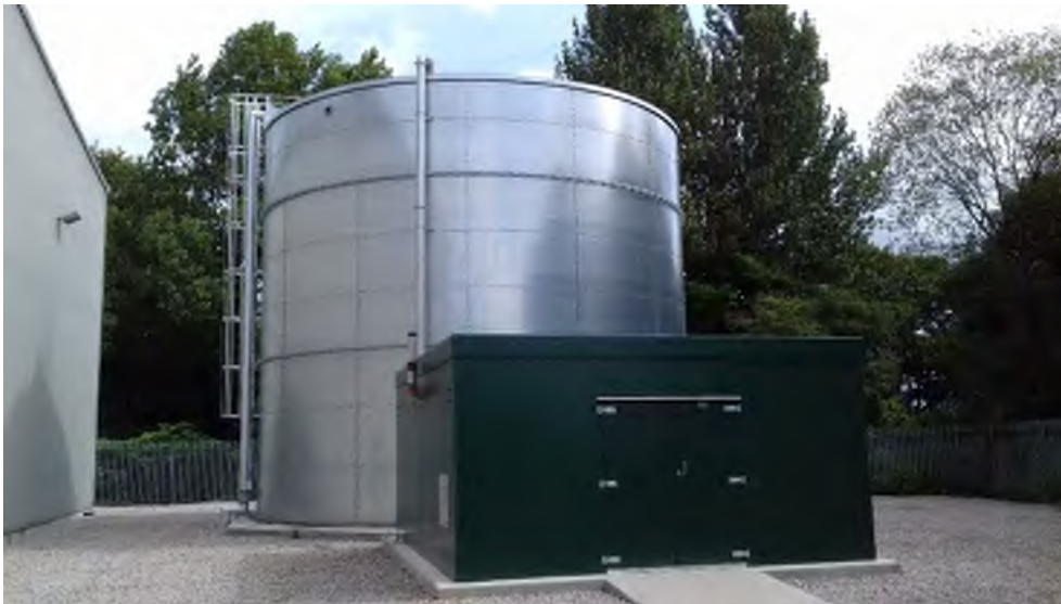
Figure 4.1 Example image of above-ground fire water tank and GRP pumping station building
