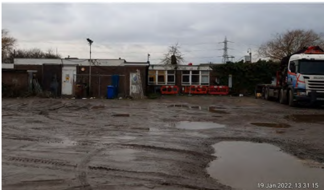
Figure 2.4 Standing flood water in semi-impermeable hardstanding
