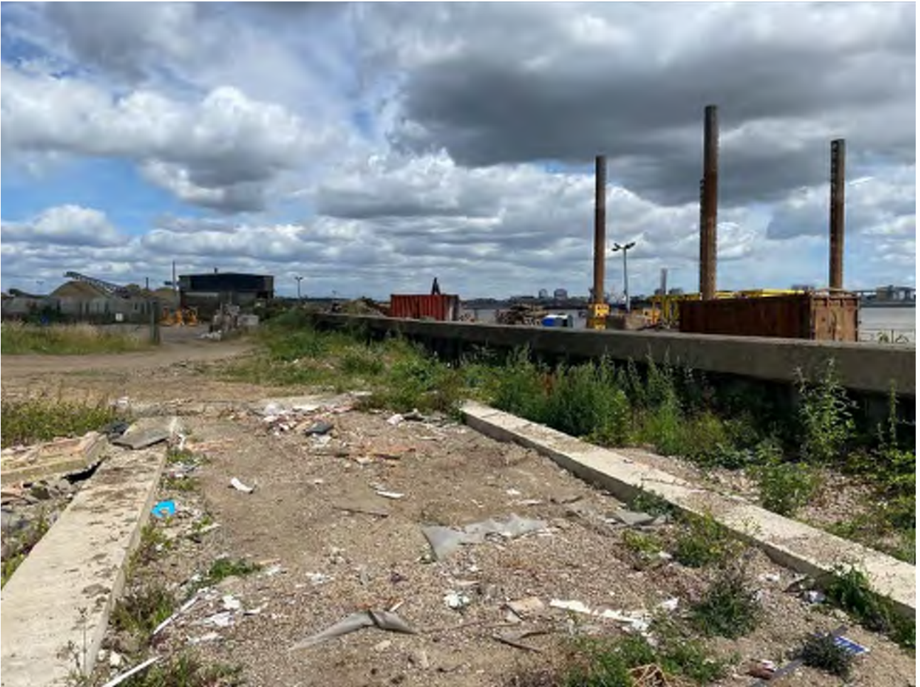
Photograph 5 Existing site and floodwall, looking north
