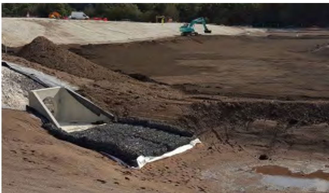
Figure 3.3 Example Reno mattress to headwall
