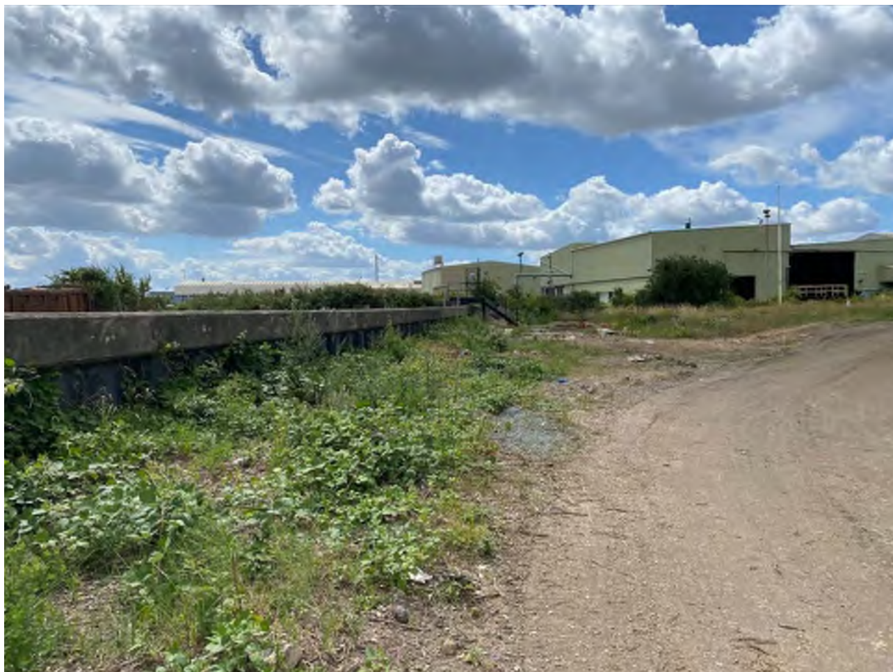
Photograph 4 Existing site and floodwall, looking south (b)
