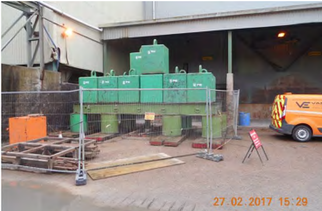
Plate 6.2 Static load test set up
