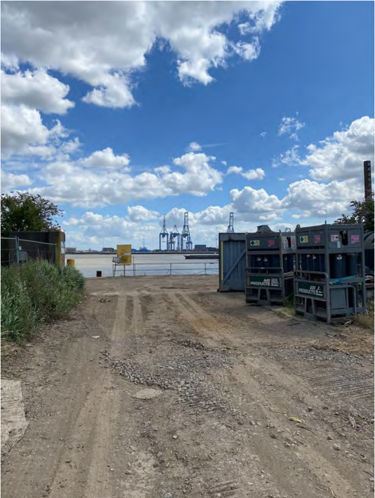
Photograph 2 EA flood gate (Asset ID: 330355)
