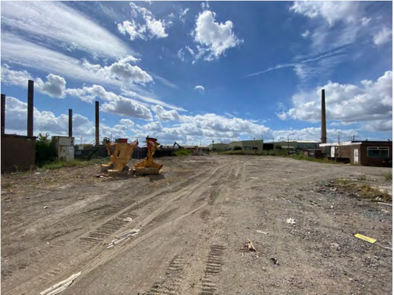
Photograph 3 Existing site and floodwall, looking south (a)
