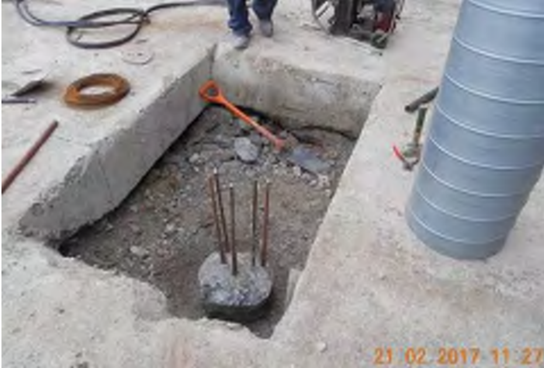
Plate 6.1 Exposed pile head and reinforcement
