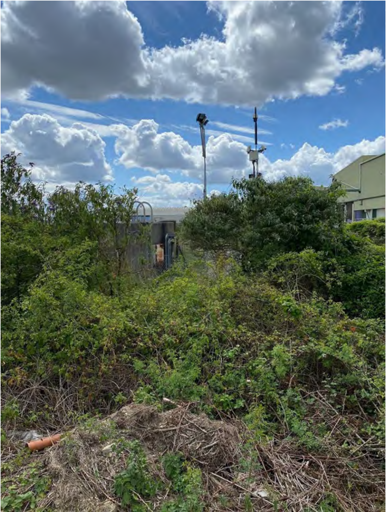
Photograph 6 EA flood gate (Asset ID: 330356)
