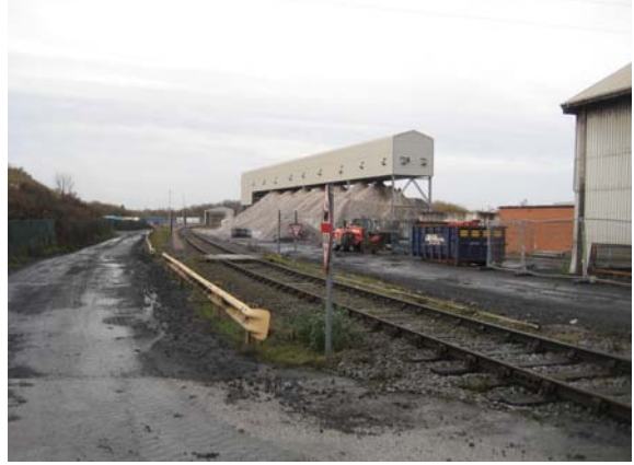
Photograph 6. Railway line and adjacent limestone store.
