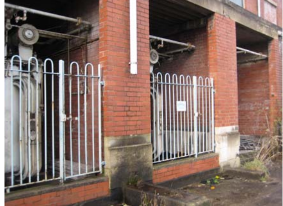
Photograph 2. Disused transformers at rear of the former power station
