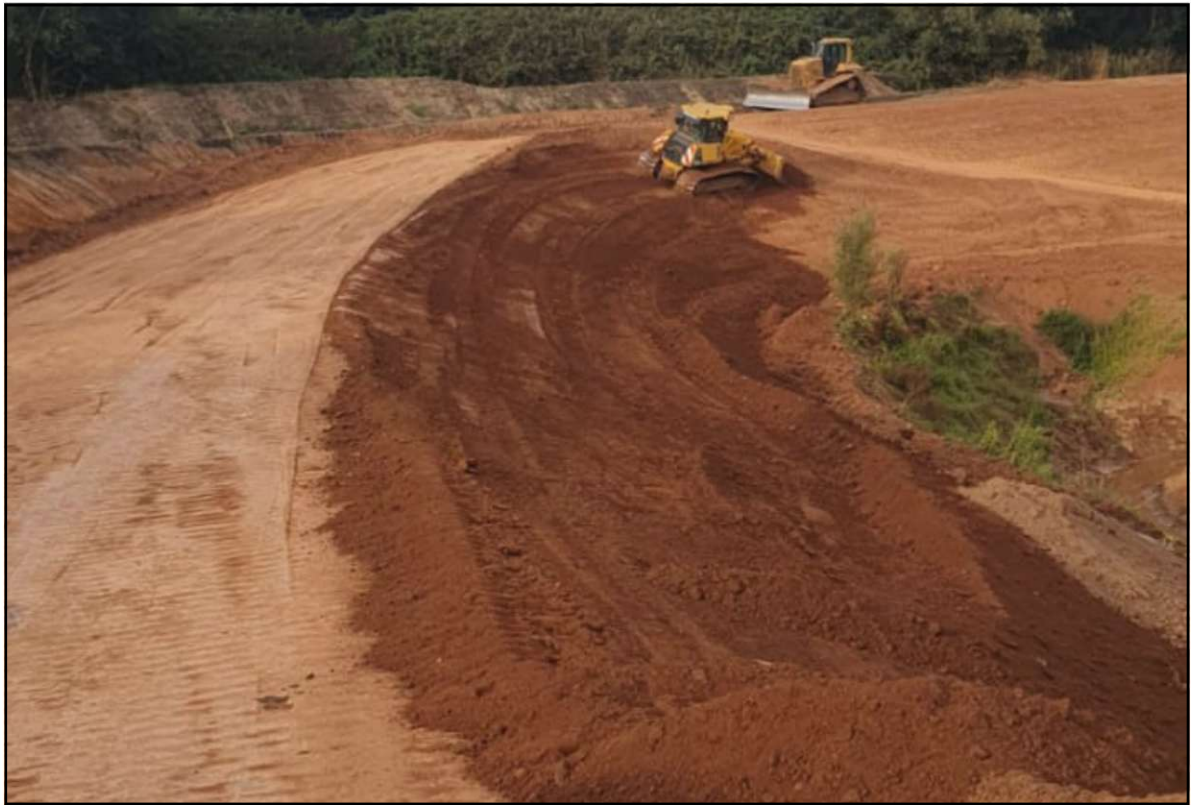
Photo 1. Material placement prior to wetting
