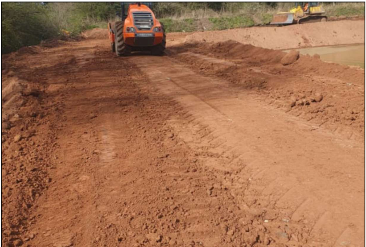
Photo 2. Material compaction
