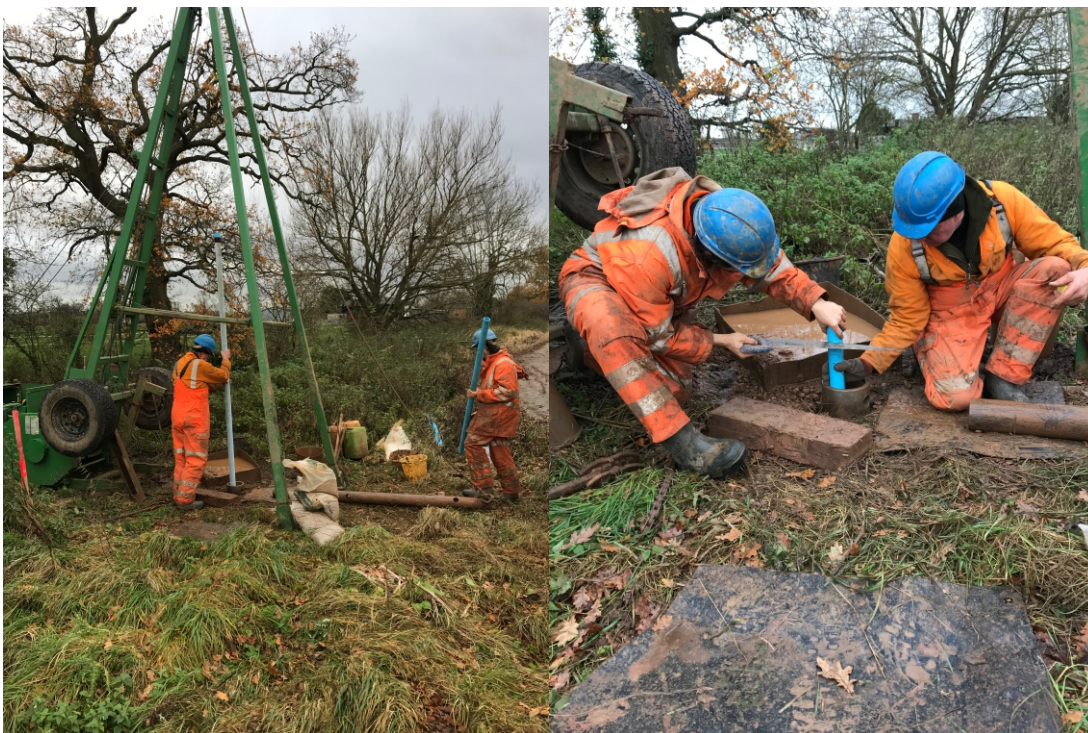
Plate 2: Inserting plain and slotted pipework to borehole annulus and cutting down to length
