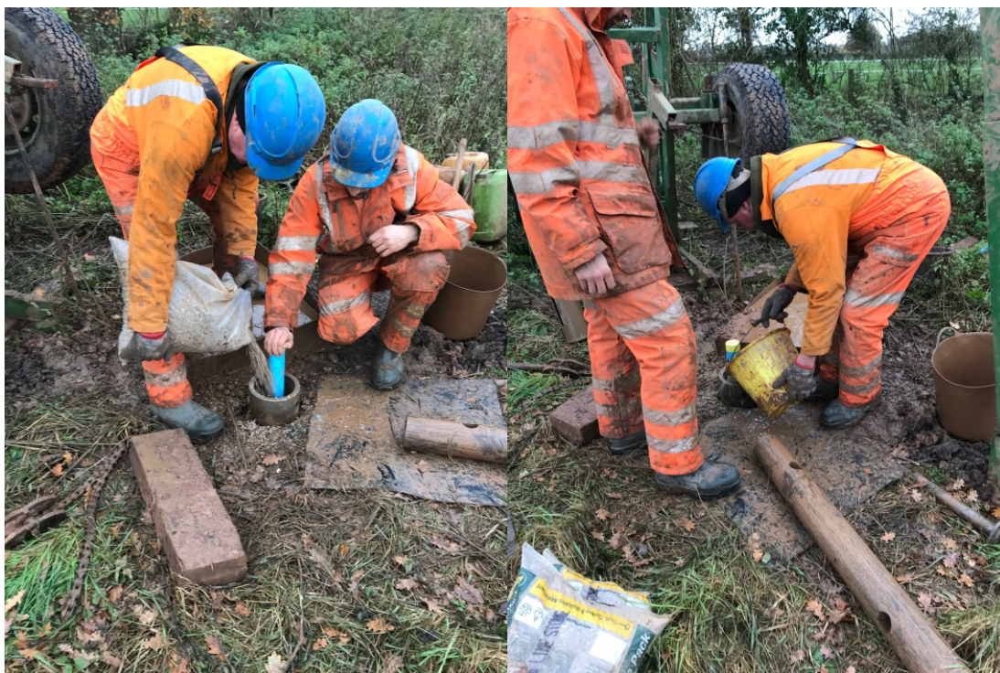
Plate 3: Backfilling with pea gravel and hydrated bentonite pellets
