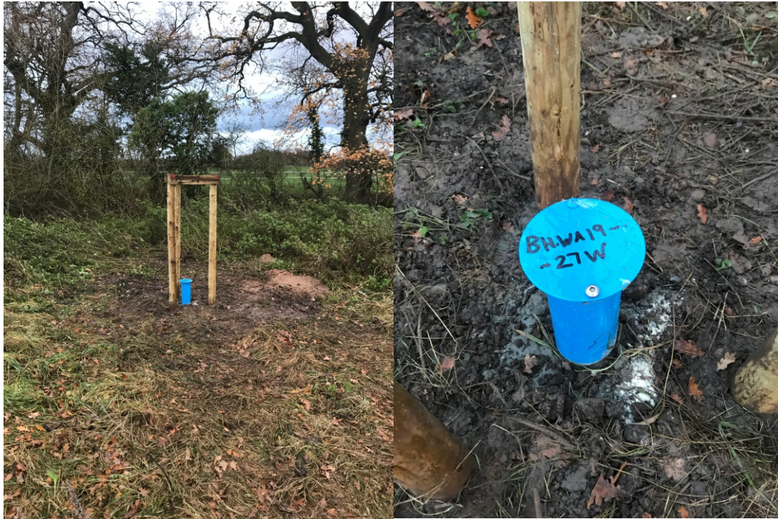
Plate 5: Installing wooden marker posts and labelling headworks with borehole reference
