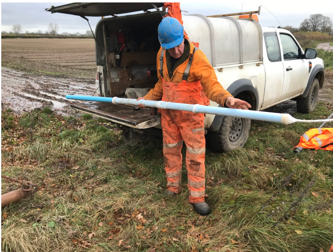
Plate 1: Covering slotted pipework with geowrap
