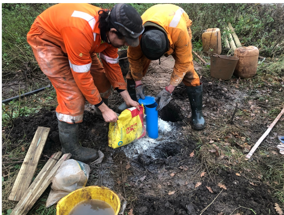
Plate 4: Cementing steel headworks in place
