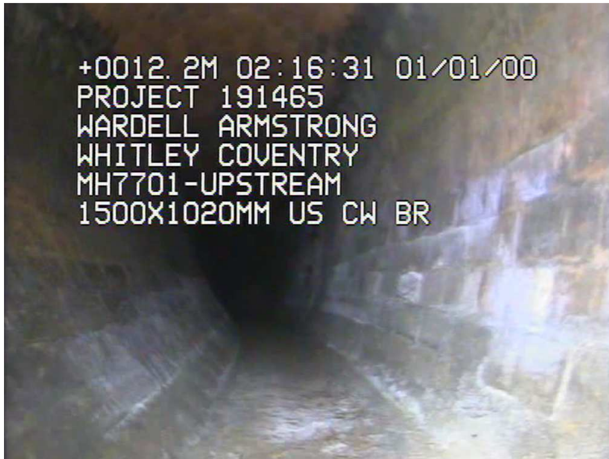
Channel upstream of MH7701 is dry with no incoming flows
