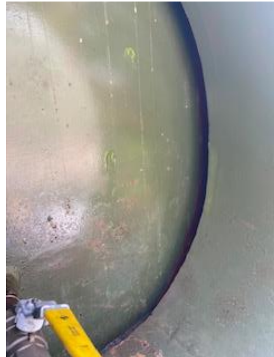
Showing inner wall surface condition.
