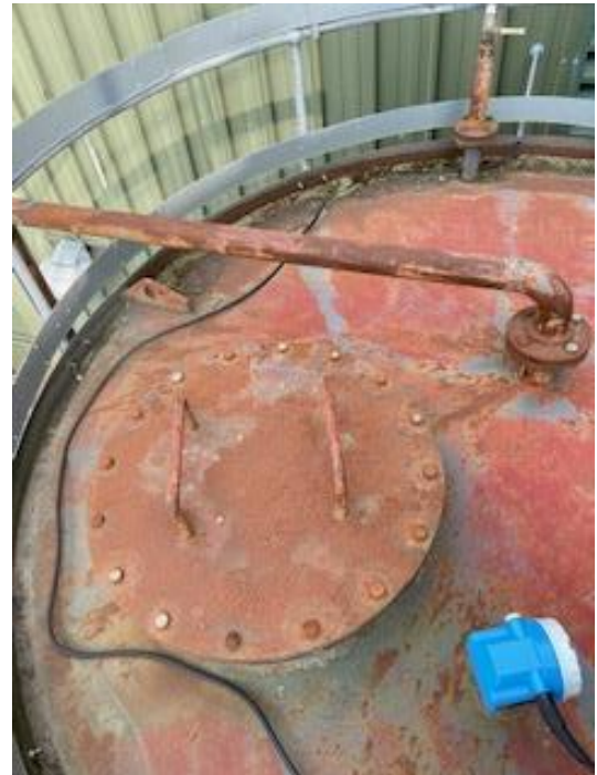
Showing roof nozzles and top manway N2.
